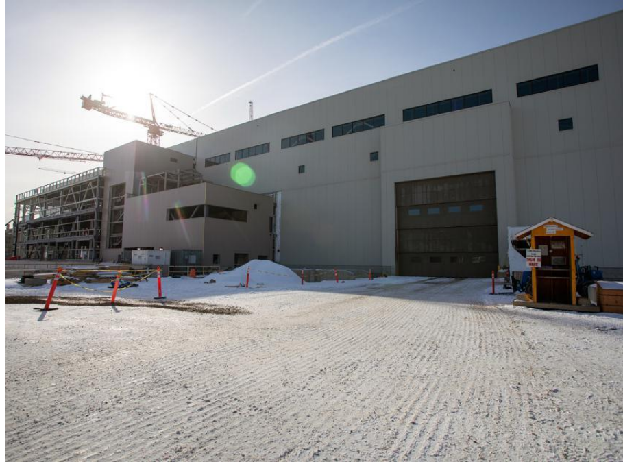
Figure A-11 Main service bay and operations building (March 2021)
