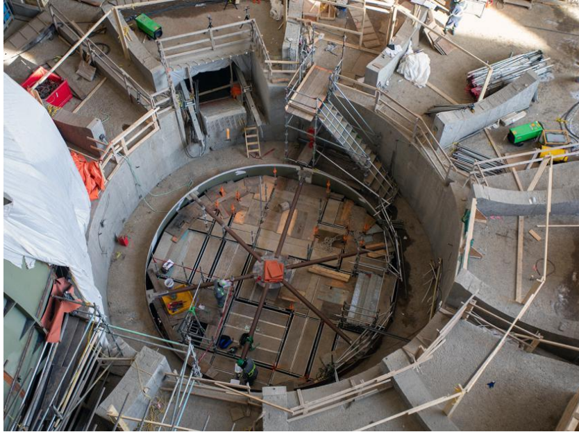
Figure A-9 Crews install the Unit 2 turbine pit elbow liner (March 2021)
