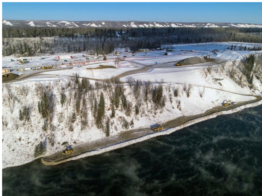
Figure A-4 Construction of the shoreline protection at Hudson's Hope (January 2021)
