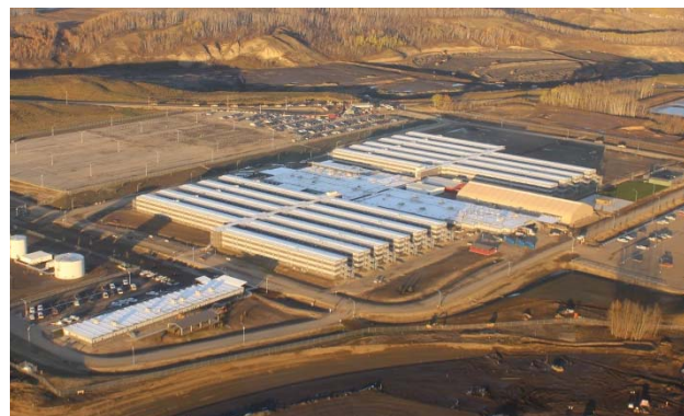
Aerial view of the worker accommodation lodge
