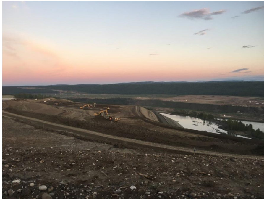
Figure A-2 Left Bank Excavation. Photo taken July 1, 2016
