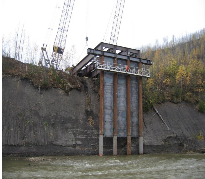
Figure A-11 Pier 1 Girders Complete for Moberly River Construction Bridge
