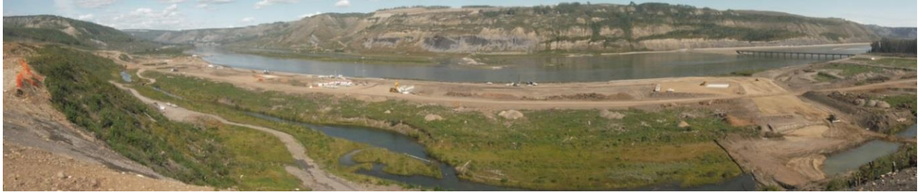
Figure A-9 Right Bank Cofferdam. Photo taken August 16, 2016
