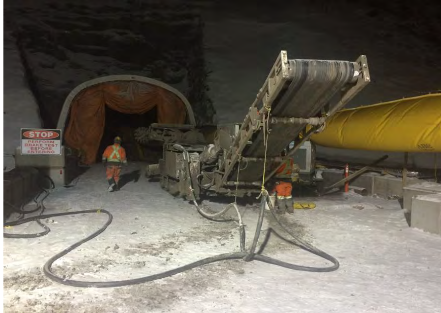
Figure A-11 Right Bank Tunnel. Photo taken March 17, 2017.
