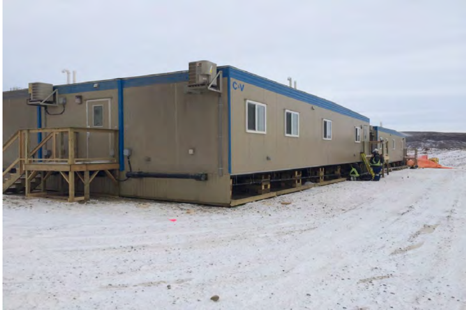
Figure A-3 Area 21 - Facing North; Continue Setting up BC Hydro Field Office. Photo taken February 11, 2017.
