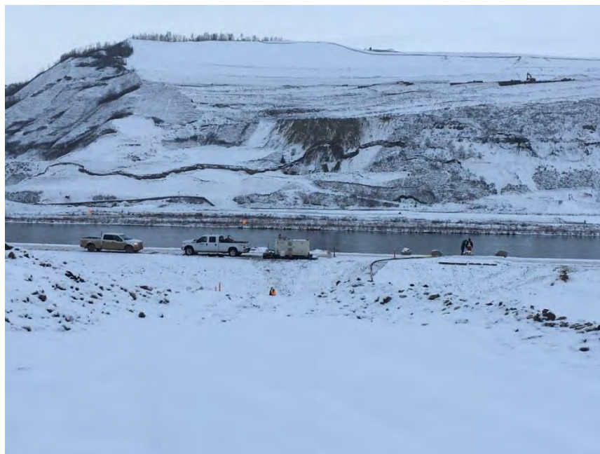
Figure A-6 North Bank Tension Crack. Photo taken February 20, 2017.
