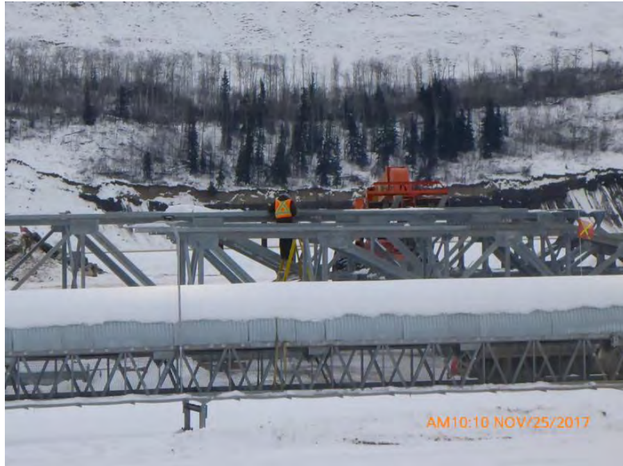
Figure A-7 Roller Compacted Concrete Conveyor Assembly. Photo taken November 25, 2017.
