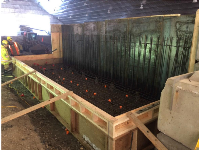
Figure A-5 Area 21, Roller-Compacted Concrete Trial Enclosure. Photo taken December 2, 2016
