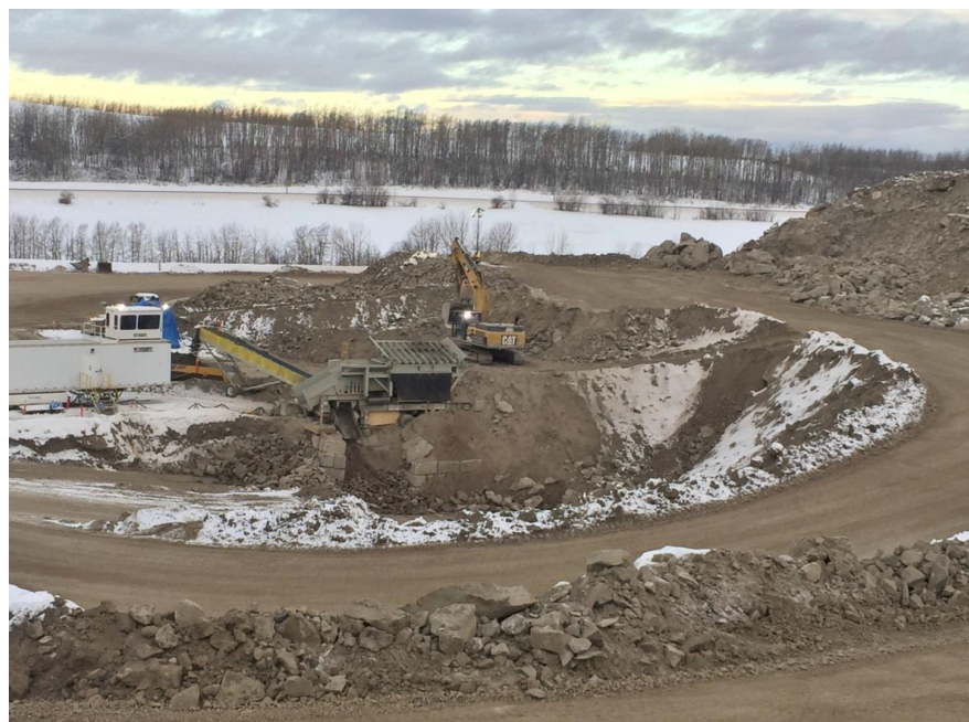
Figure A-10 Wuthrich Quarry Facing West – Plant Layout. Photo taken December 2, 2016
