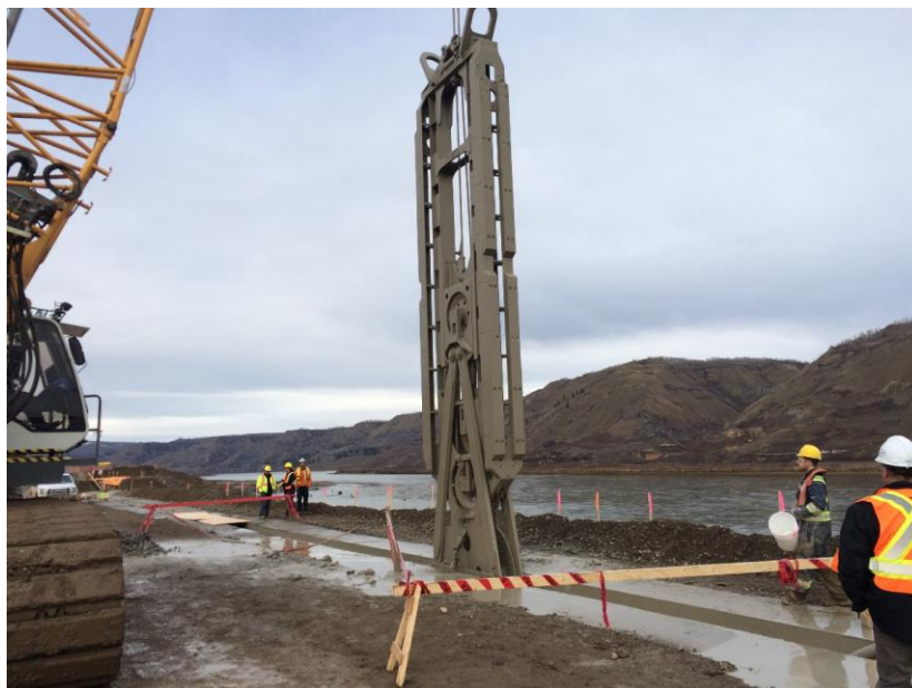
Figure A-2 Right Bank Cofferdam – Grab 2 Installing Panel 246. Photo taken November 5, 2016
