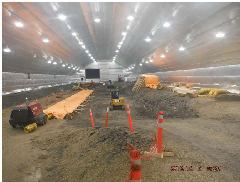
Figure A-8 Roller-Compacted Concrete Trial Enclosure. Photo taken December 2, 2016
