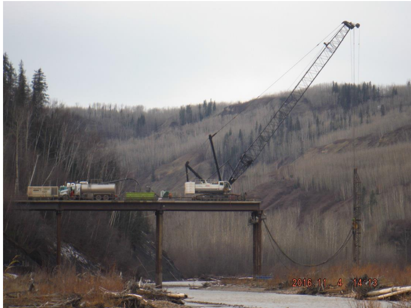
Figure A-1 Moberly River Construction Bridge Facing South. Photo taken November 4, 2016.
