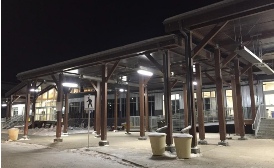
Figure A-11 Worker Accommodation North Mud Room and Lobby Entrance.
