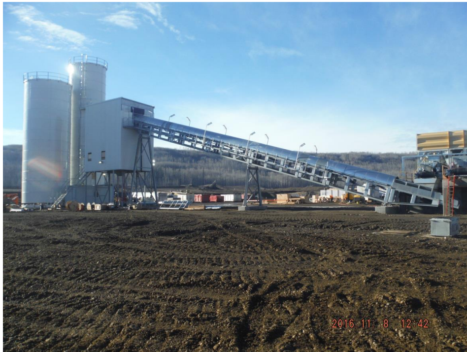
Figure A-4 Commissioning Concrete Plant. Photo taken November 8, 2016
