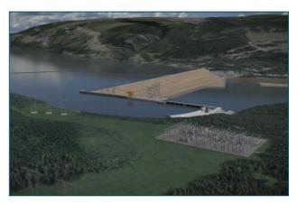
A new Site C substation will be constructed near the Site C dam on the south side of the Peace River. The substation will connect the power feed from the Site C generating station to the new 500 kV lines and the supply to Fort St. John and Taylor.
