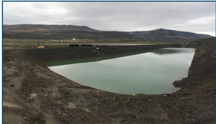
Above: Sediment pond at the Site C dam site. Sediment ponds are a best practice in sediment control. During a rain event, these ponds capture runoff that may contain eroded soil. The pond allows the sediment to drop to the bottom and keeps the water exiting the pond clean.
