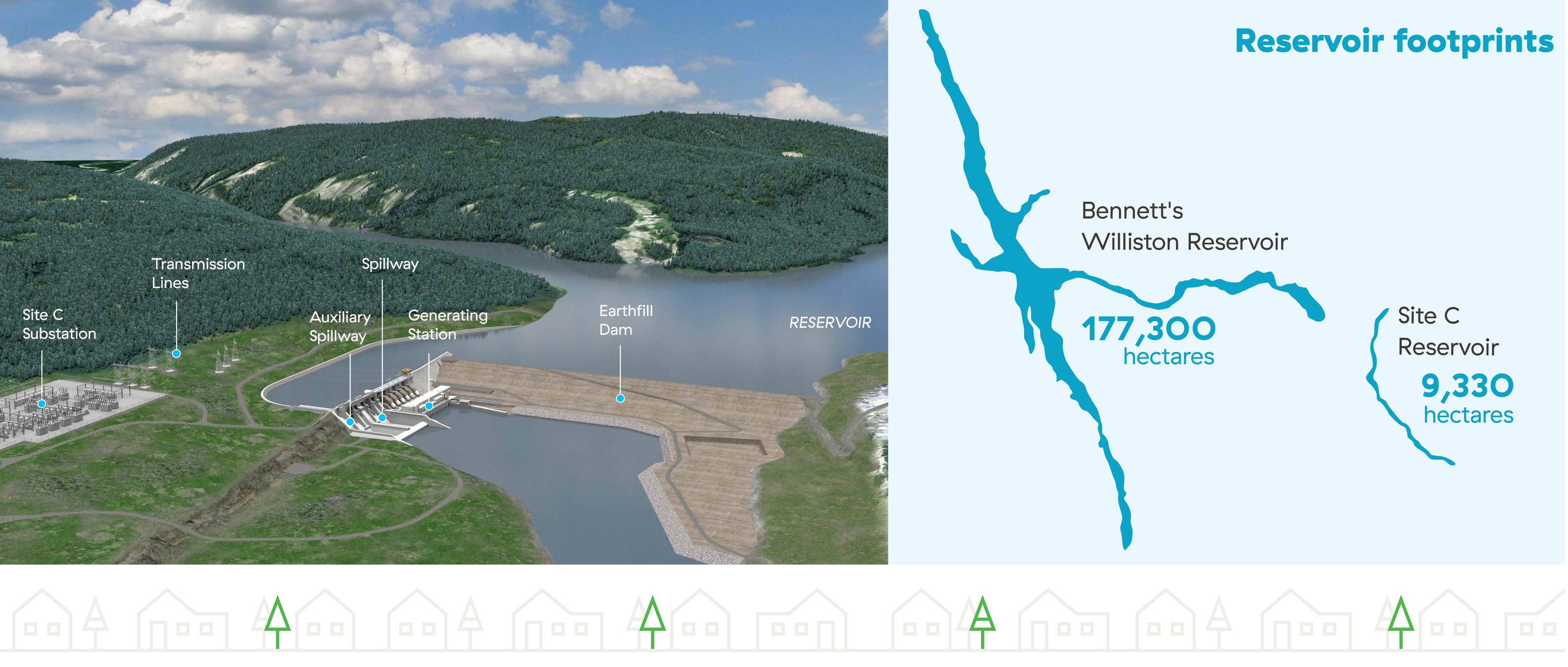
The Site C project builds on BC Hydro's existing system. Because it uses water already in the Williston Reservoir, Site C will generate 35% of the electricity of the WAC Bennett Dam, using a reservoir only 5% of the size. Once it is built, the Site C generating station will produce 5,100 gigawatt hours of clean electricity every year, enough to power 450,000 homes in B.C.
