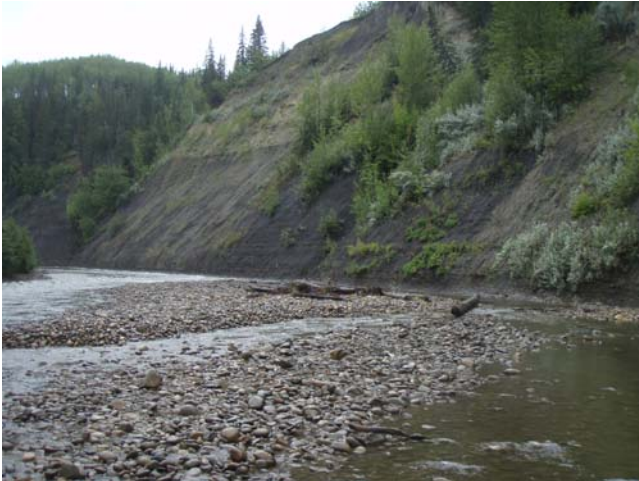
Plate 7 Zone 4. Example of valley wall erosion on the Moberly River, 2009.
