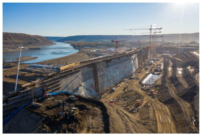
Crews are removing the temporary ramp used to construct the dam and core buttress, and they are installing insulation on the upstream side of the buttress. See more project photos in the <u>image gallery</u>.
