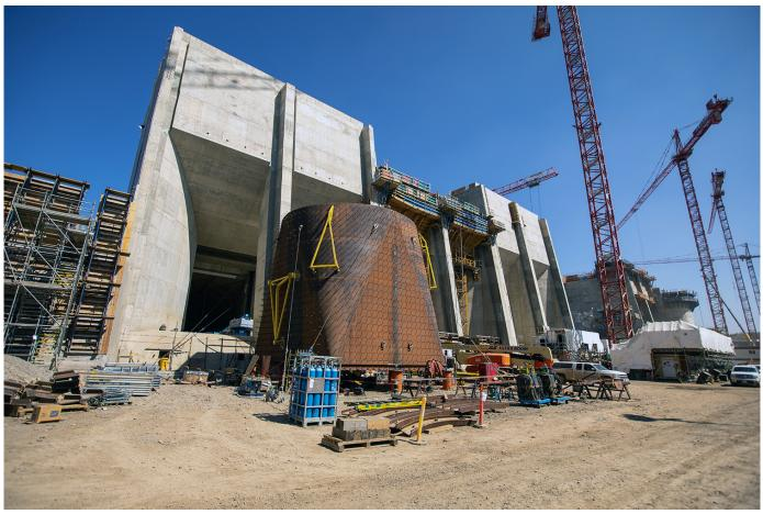
Intake units 1 and 3 are substantially complete, with unit 2 under construction. The unit 4 penstock transition piece is pictured in the foreground. See more project photos in the <u>image gallery</u>.
