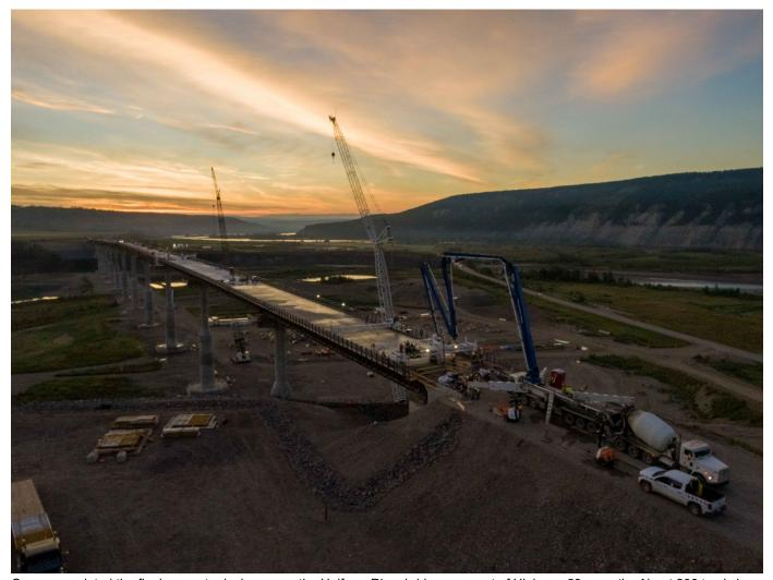
Crews completed the final concrete deck pour on the Halfway River bridge segment of Highway 29 recently. About 200 trucks' worth of concrete was placed on the one-kilomtre bridge deck in 13 pours.
