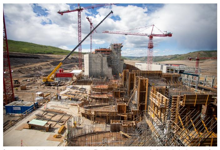
Crews are constructing the upper spillway headworks. The spillways are an important safety feature, allowing the passage of large volumes of water from the future reservoir into the river channel downstream. See more project photos in the  $\underline{\mathsf{image gallery}}$ .
