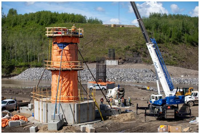
Crews have begun pouring concrete to build the piers for the Cache Creek bridge as part of the Highway 29 realignment. The bridge will have six piers, and the bridge will be 44 metres tall at the highest point. See more project photos in the <u>image gallery</u>.
