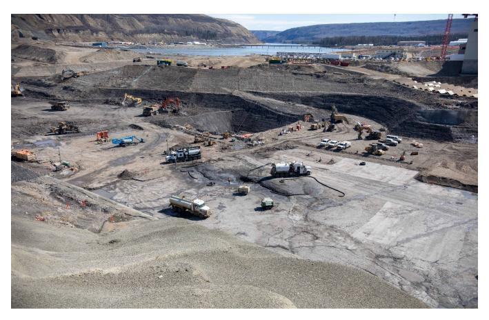
Crews excavate and prepare the dam core area where the earthfill dam will be constructed. See more project photos in the <u>image gallery</u>.
