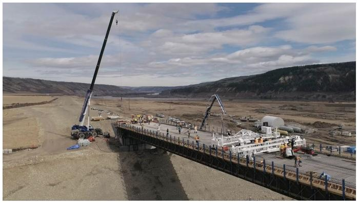
Crews completed the first concrete placement pour on the Highway 29 Halfway River Bridge deck recently. Concrete was placed using a concrete pump truck and then levelled with a screed machine, which moves on rails to level the concrete to the correct thickness and slope for the deck. See more project photos in the <a href="mailto:image gallery">image gallery</a>.
