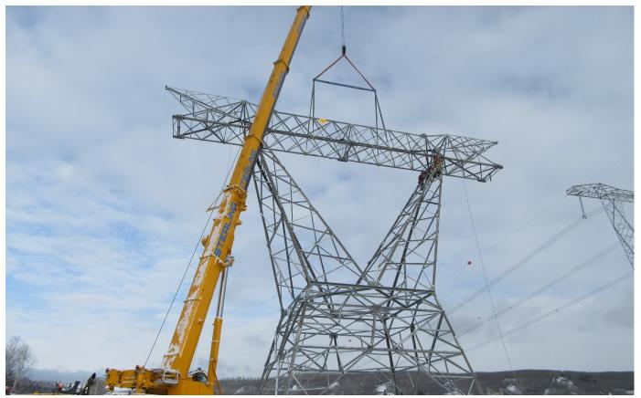
The last of 205 transmission towers on the second transmission line was completed at the end of March. Stringing will begin later this summer, and when finished, the new line will connect the Peace Canyon substation to the Site C substation. See more project photos in the <u>image gallery</u>.
