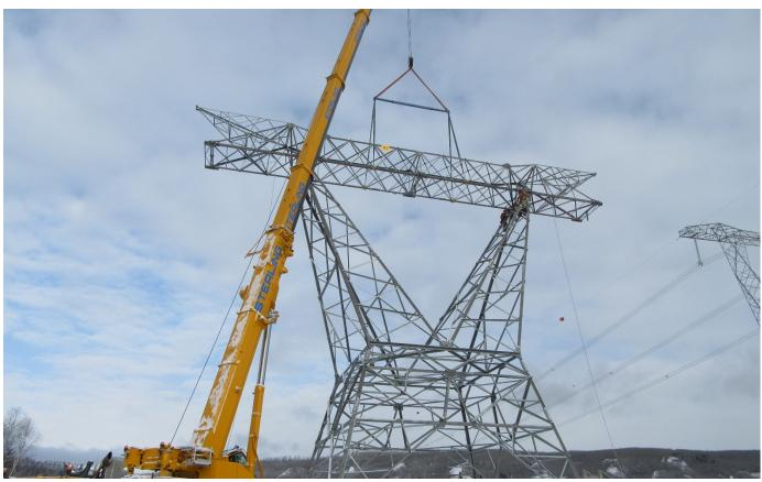
The last of 205 transmission towers on the second transmission line was completed at the end of March – eight months ahead of schedule. Stringing will begin later this summer, and when finished, the new line will connect the Peace Canyon substation to the Site C substation. See more project photos in the <u>image gallery</u>.
