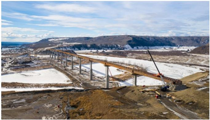
Crews completed installing the steel bridge girders – the main horizontal support beams – across the Halfway River bridge. The girders were assembled in 27 sections with 81 separate pieces. See more project photos in the <u>image gallery</u>.
