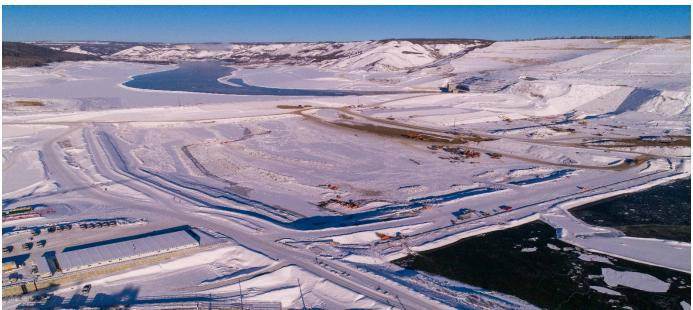
The upstream cofferdam was recently completed to its final elevation, approximately 24 metres high above the riverbed. The upstream and downstream cofferdams seal off the Peace River and direct water through two diversion tunnels. See more project photos in the <u>image gallery</u>.
