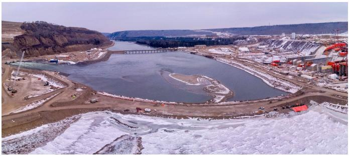
An aerial view of the downstream cofferdam. Both the upstream and downstream cofferdams have been installed across the river and interlocking steel pile walls have been completed. See more project photos in the <u>image gallery</u>.
