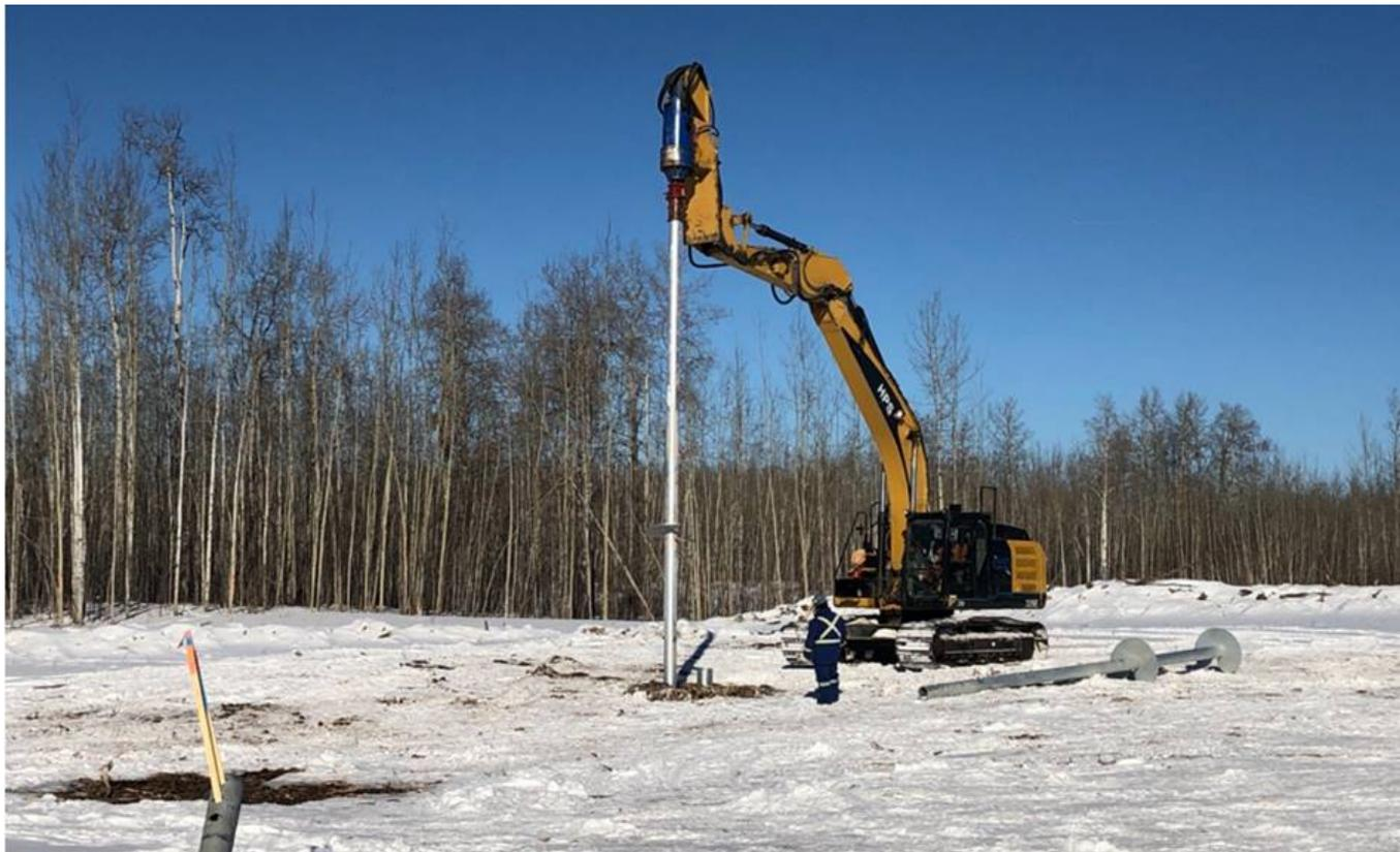
The helical piles are tall steel pipes with a screw at the bottom (the helix). The pipes are twisted deep into the ground, pull tested to confirm their strength, and a steel cap is welded on top before the transmission tower is placed above. Overall, 3,800 helical piles have been installed.
