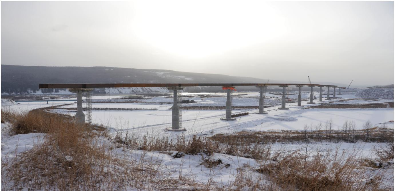
All twelve bridge piers for the Halfway River are now complete and steel girders are being installed on top. In this area, the reservoir will cover the existing highway and bridge, requiring re-alignment of the highway and construction of a new bridge. This new segment of highway will be three kilometres long, and the new bridge will be one kilometre long. See more project photos in the [image gallery](#).
