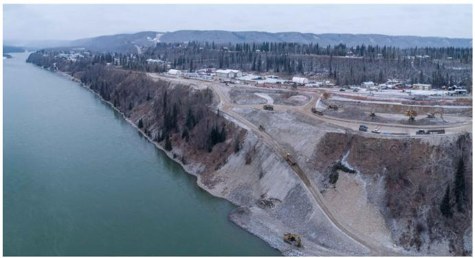
The construction of a 2.6-kilometre-long berm to protect the shoreline of Hudson's Hope is underway. See more project photos in the <u>image gallery</u>.
