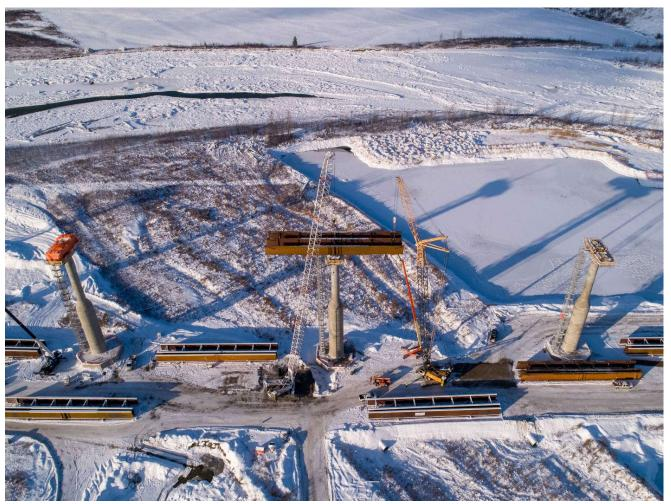
The first steel girder was installed at the Halfway River Bridge on November 18, 2020. See more project photos in the <u>image</u> <u>gallery</u>.
