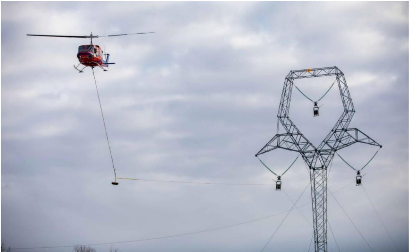
Helicopters are used to string the sockline between the transmission towers. See more project photos in the [image gallery](#).
