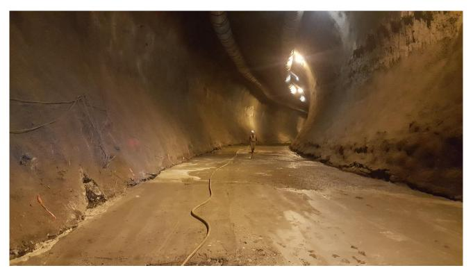
In late December 2019, we substantially completed excavations in the two Peace River diversion tunnels. The tunnels are temporarily coated with shotcrete until the permanent concrete liner is installed. See more project photos in the <u>image gallery</u>.
