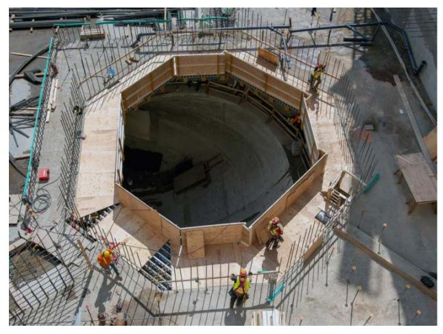
View of the inside of a draft tube in the powerhouse. Once Site C is operational, water will enter the penstocks and move through the turbines and generators, and then be released into the draft tubes before exiting through the tail race into the Peace River. See more project photos in the <a href="mage-gallery">image-gallery</a>.
