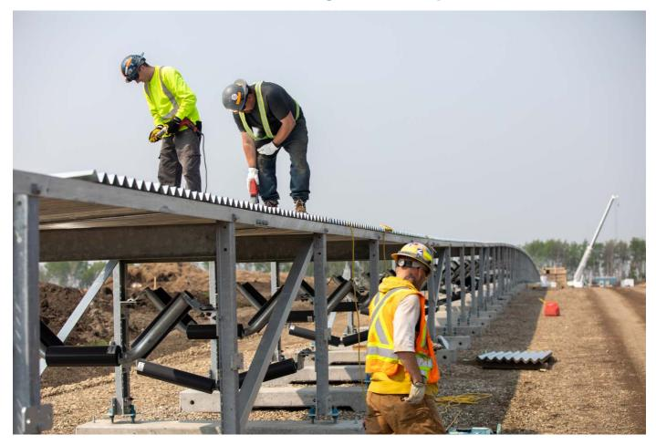
Workers install overhead cladding to protect the till conveyor belt. See more project photos in the image gallery.
