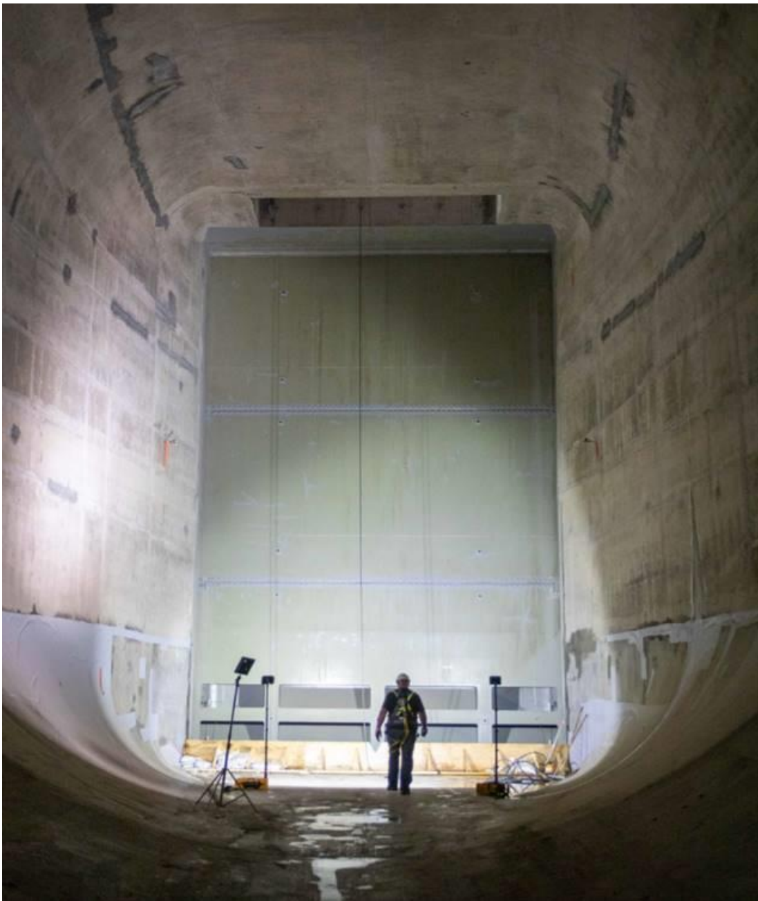
Leakage test of the Tunnel #2 gates, the water on the other side of that gate is more than 10m high.
