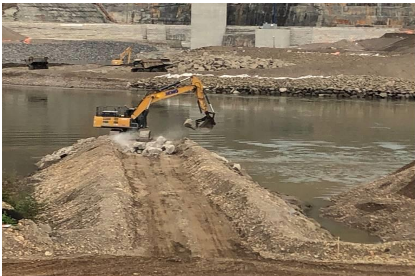
Rockberm encroachment continuing to 35 per cent.
