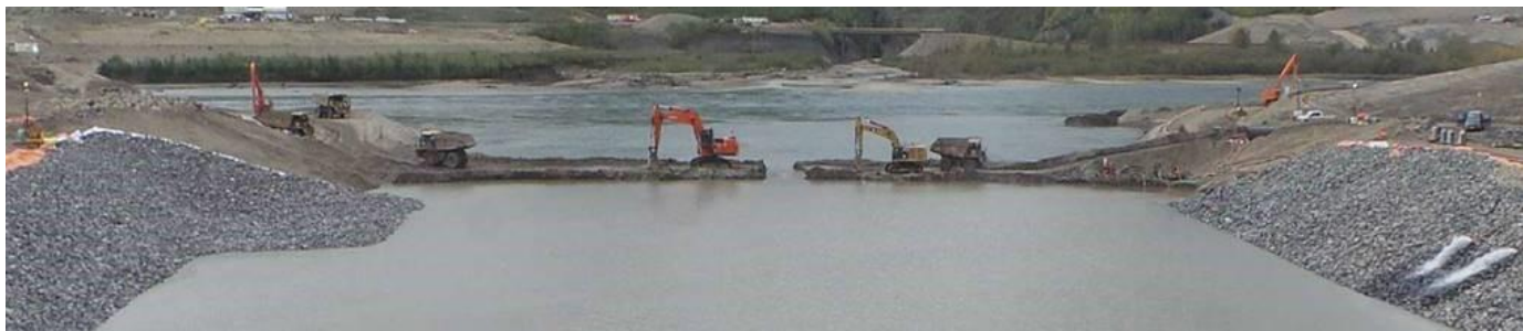
September 11, 2020 – Excavators removing material to open the cofferdam on the inlet channel.
