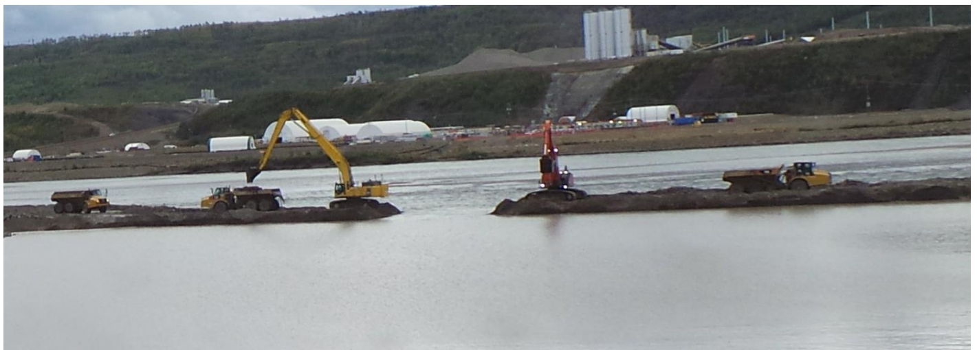
September 11, 2020 – Excavators removing material to open the cofferdam on the outlet channel.
