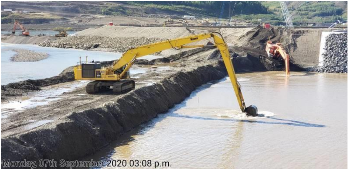
Two long boom excavators working together (one removing material, one placing rock) on the outlet channel.
