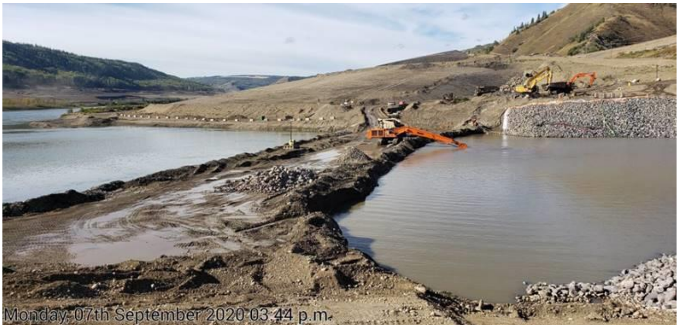
A long boom excavator placing rock armouring on the inlet channel
