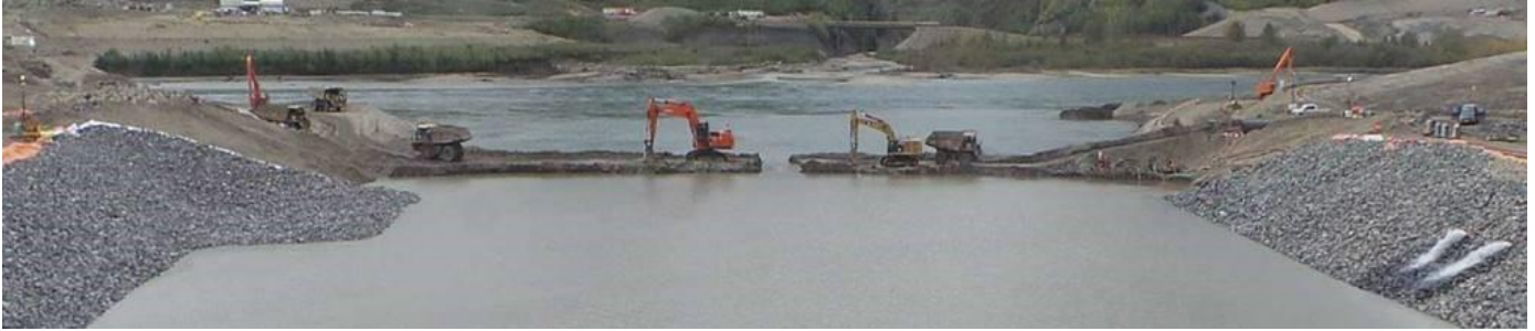
September 11, 2020 – Excavators removing material to open the cofferdam on the outlet channel.
