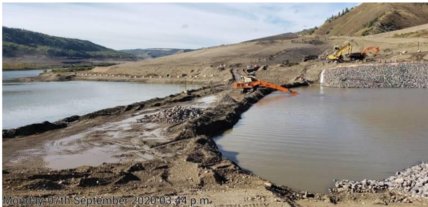
A long boom excavator placing rock armouring on the inlet channel
