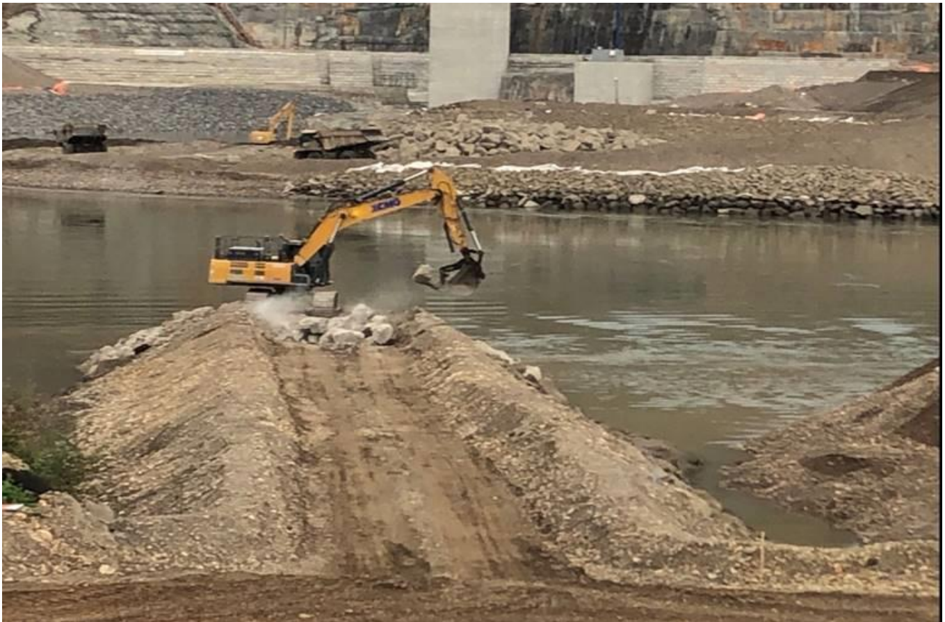
Rockberm encroachment continuing to 35 per cent.
