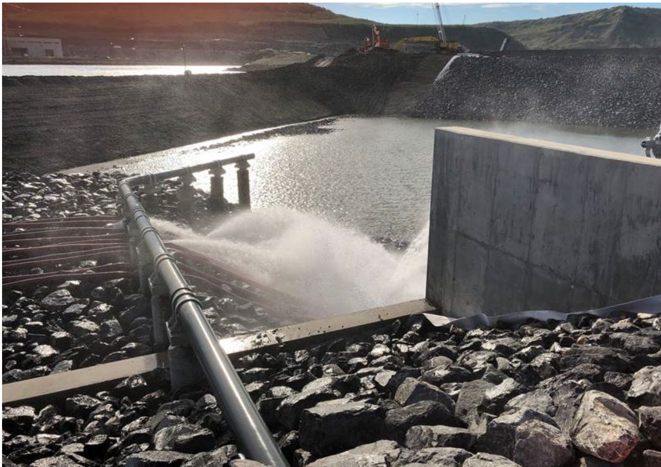
Pumping underway at the outlet channel
