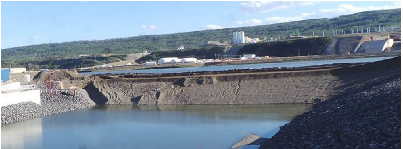
Outlet cofferdam removal progress as of August 17, 2020
