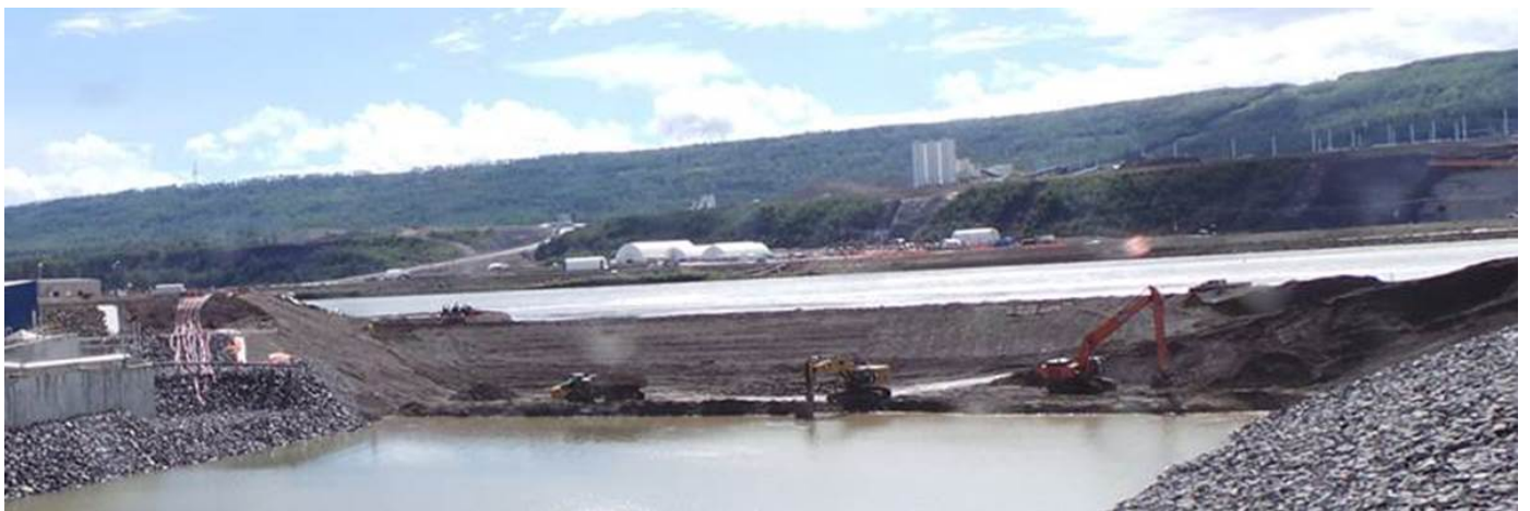
Outlet cofferdam removal progress as of August 24, 2020
