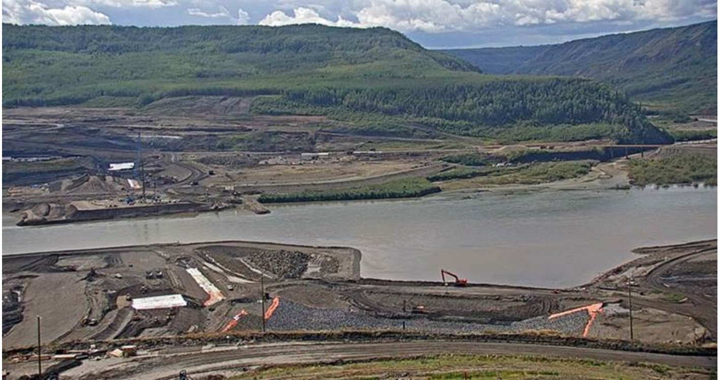
View from the north bank
