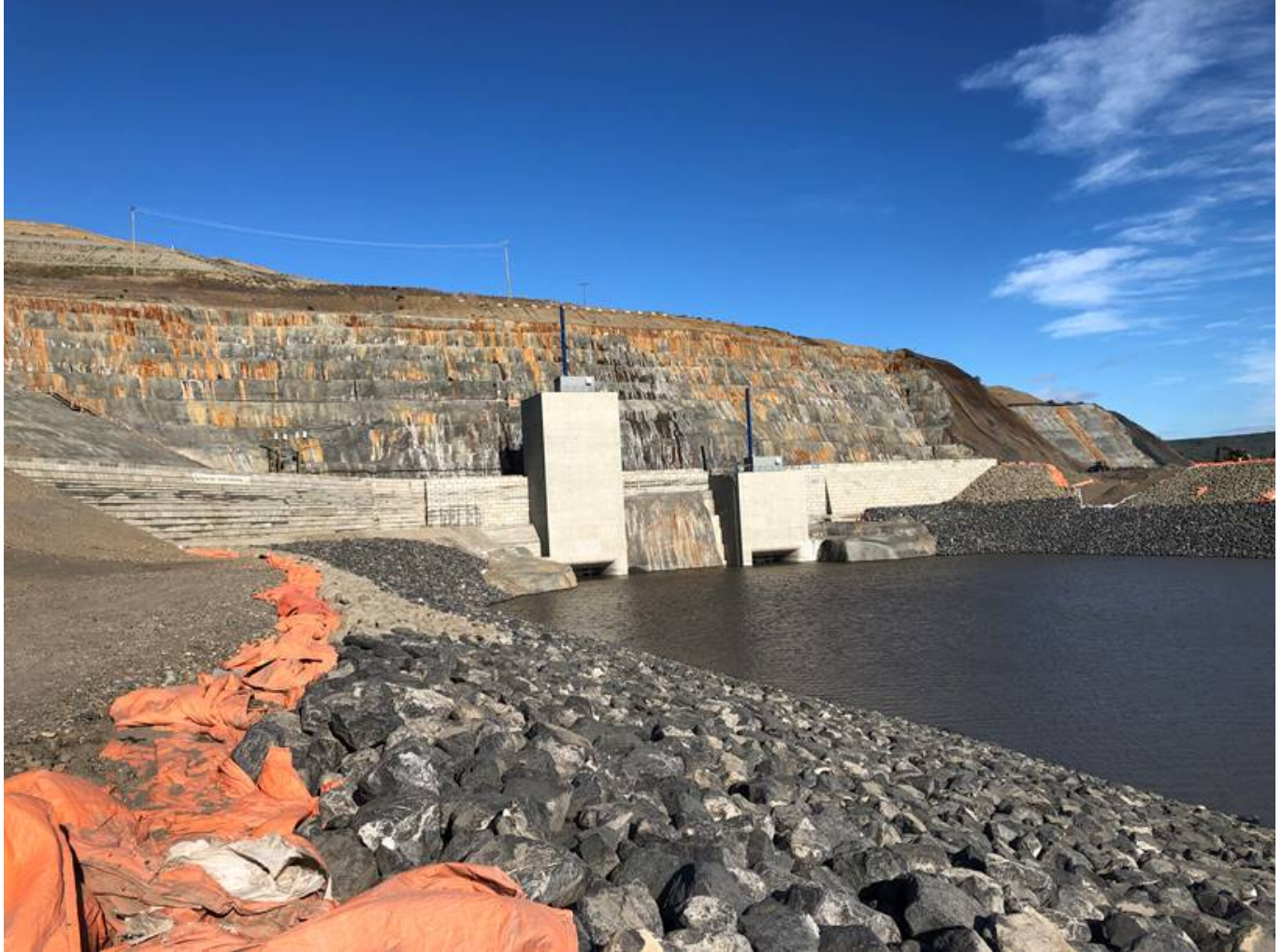
Inlet channel with pumping complete
