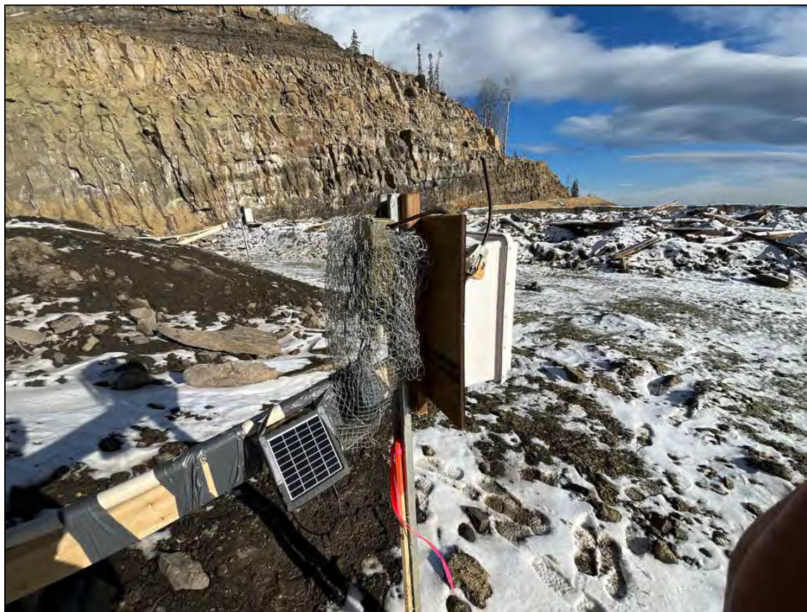
Figure 10. An ARU attached to the data collection station at hibernaculum Site 1-31 enclosed by wire mesh to prevent wildlife tampering.
