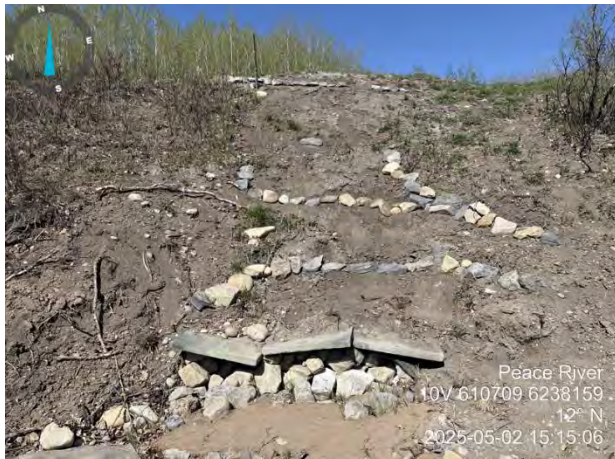
Photo 3. Rock armoring added by hand on the exposed slope above the hibernaculum. 2025-05-02.
