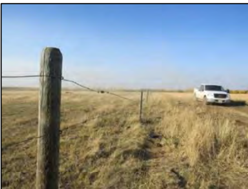
Photo 5. Existing fencing needing repair
