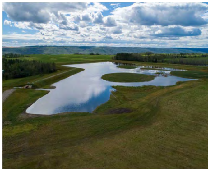
Figure 5. Golata Canyon Ranch excavated wetland (Basin 1)
