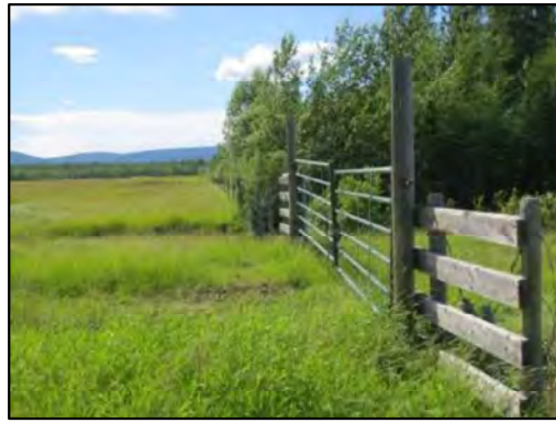
Photo 4. Existing fencing in good condition
