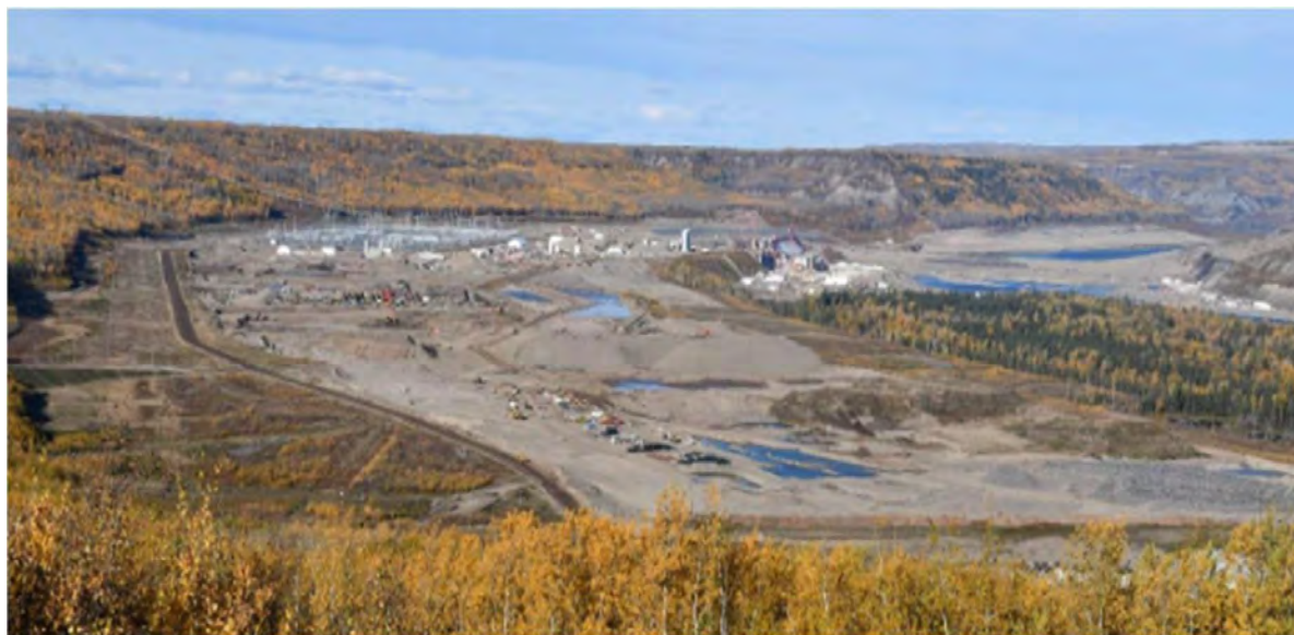
Figure 15. Area A looking west towards the Site C dam
