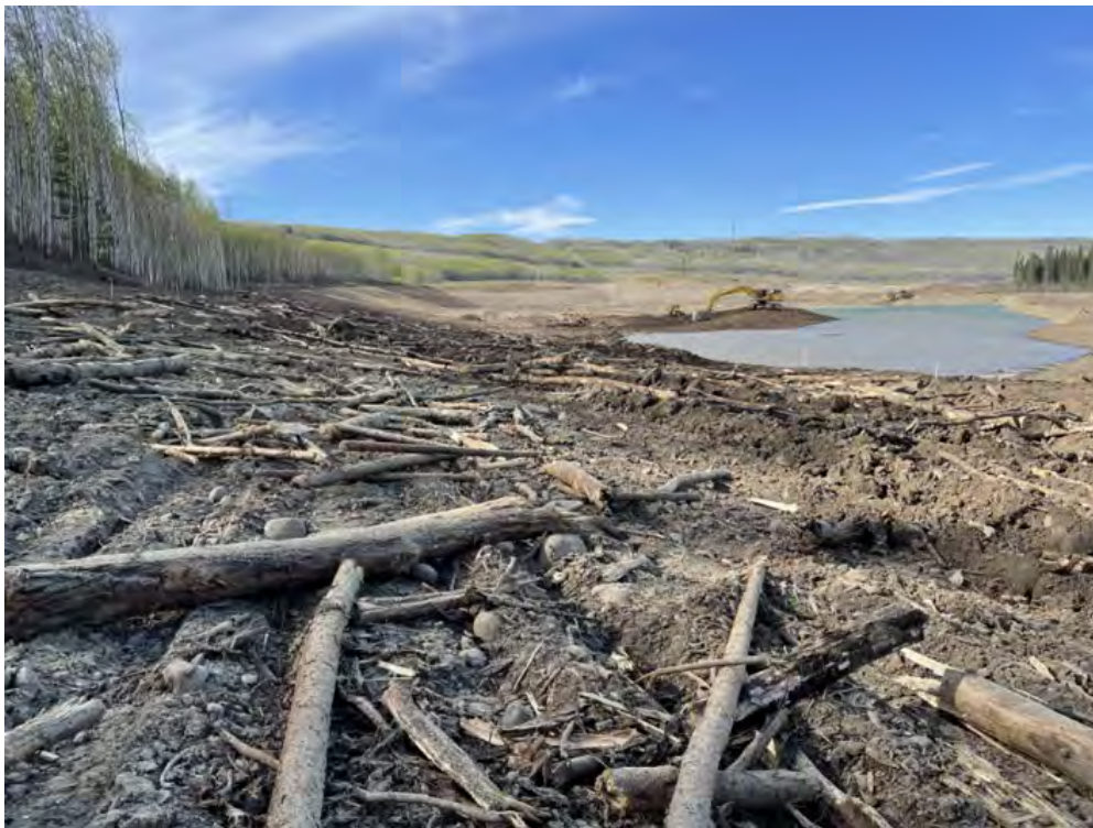
Figure 16. Physical reclamation within Area A Basins 1 – 3 which included contouring, topsoil placement, ripping and furrowing, coarse woody debris placement and native grass seeding. This photo was taken in August 2024 showing some of the woody debris placement.
