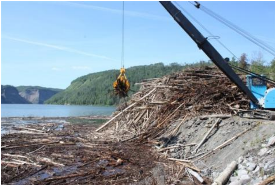
Photograph 10 Crane used to extract woody debris
