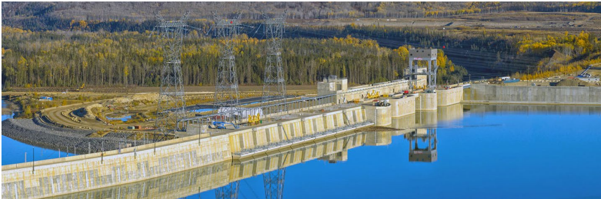
Figure A-2 Upstream side of the generating station and spillways. From the left, the dam buttress, the six generating station intakes, and the spillways on the right side. The three transmission towers sit on top of penstock units 1,3 and 5 (October 2025)
