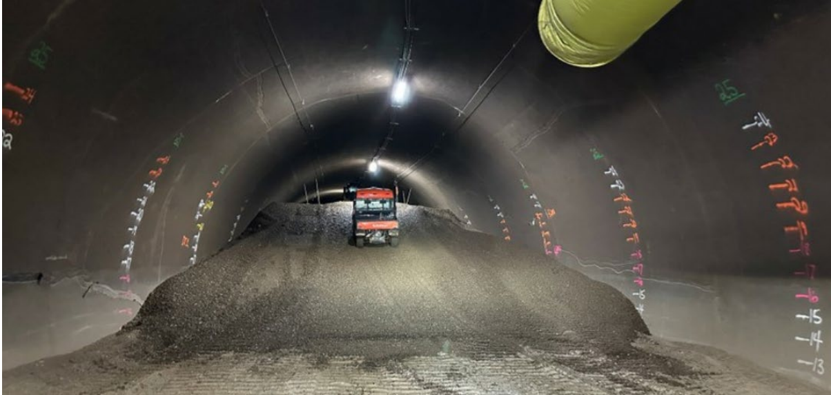
Figure A-27 Backfill of Diversion Tunnel 1 and 2 (March 2026)
