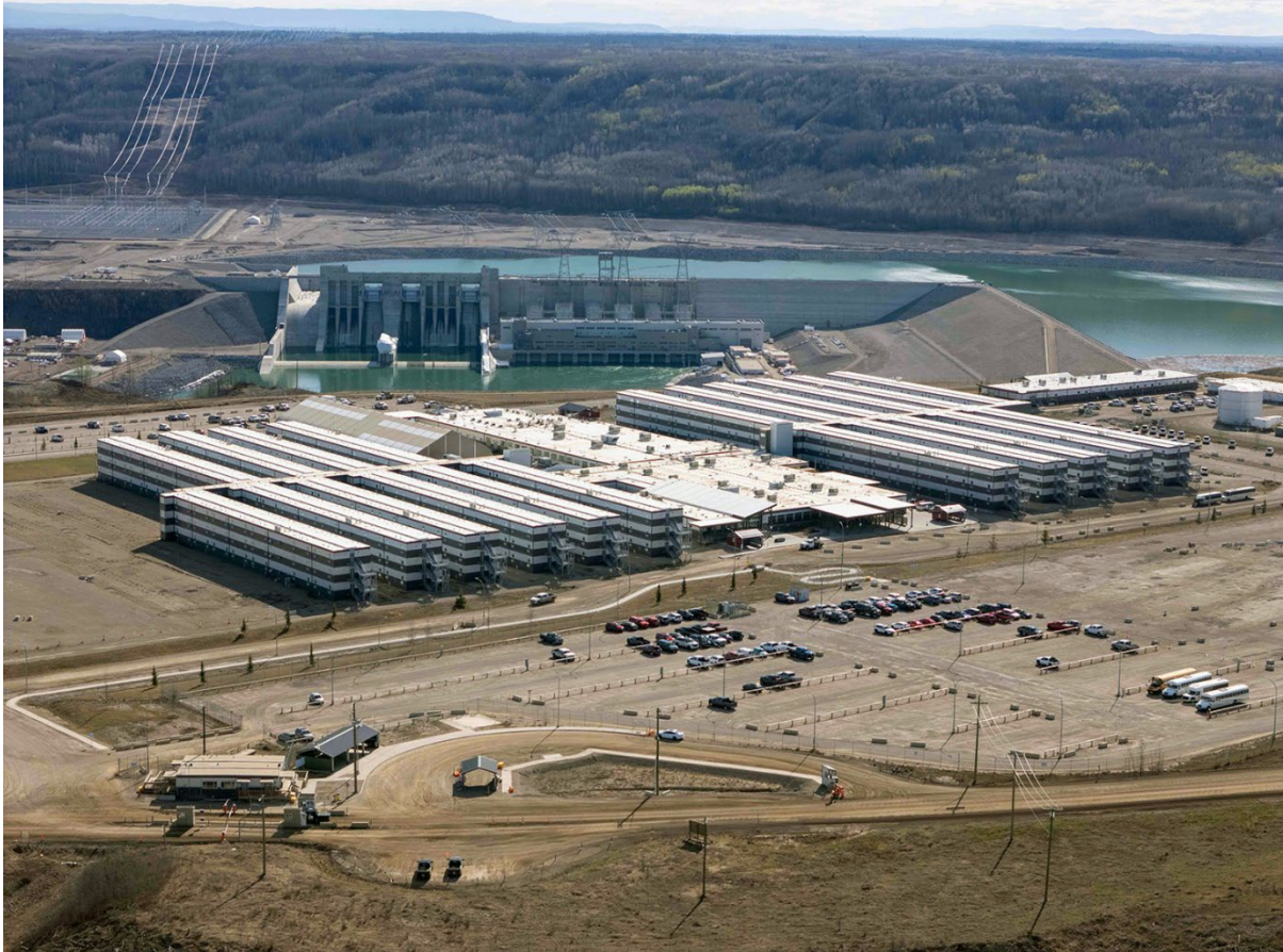
Figure A-29 Site C Worker Accommodation Camp (March 2026)
