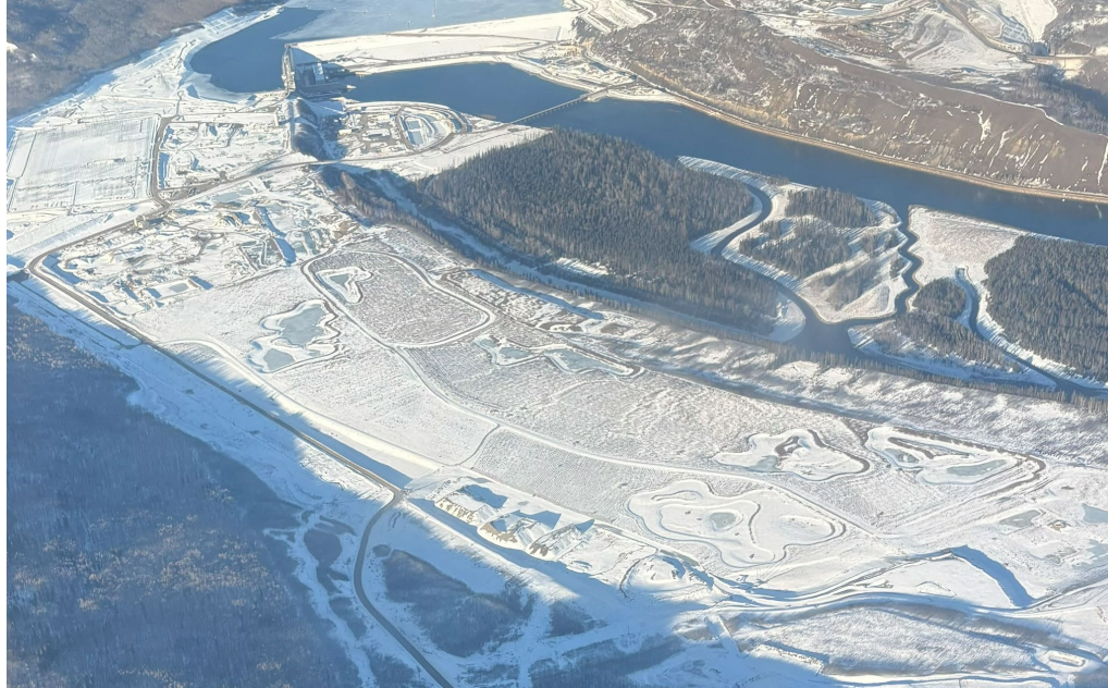
Figure A-18 Area A Reclamation (January 2026)
