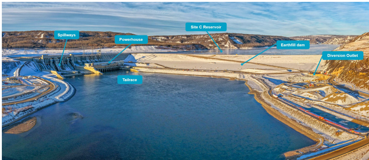
8 Figure 1 The Site C Dam Site (as seen in March 2026).
