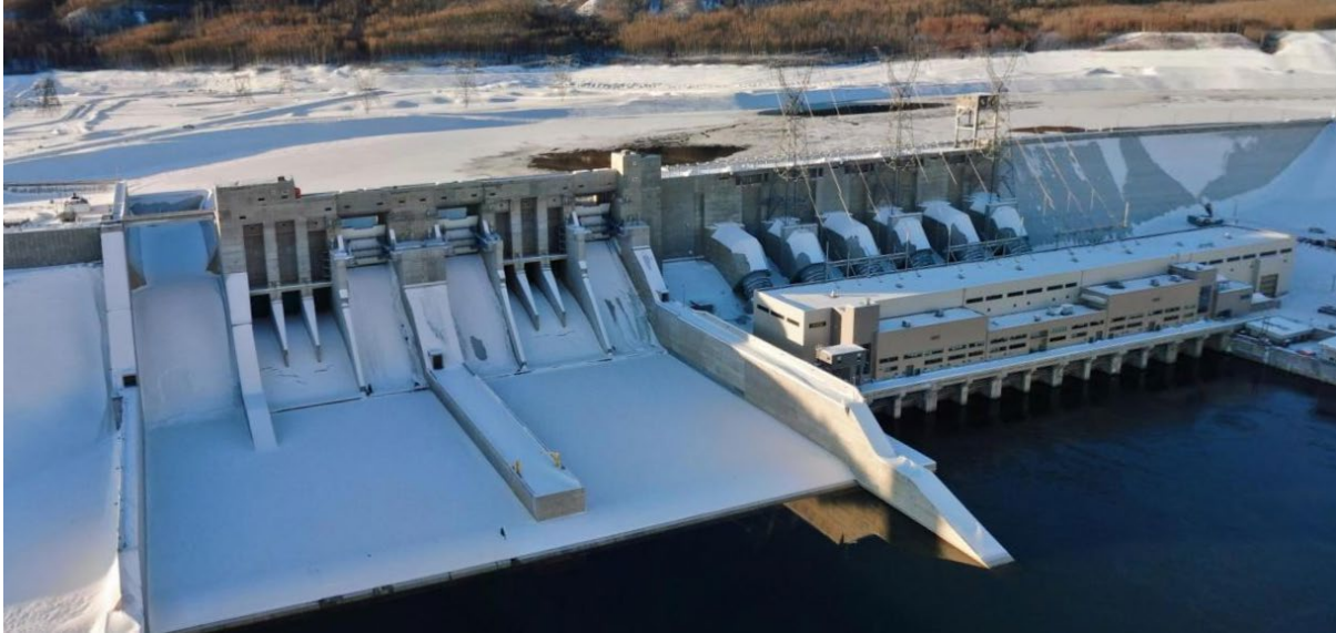
Figure A-26 Spillway and Powerhouse (January 2026)
