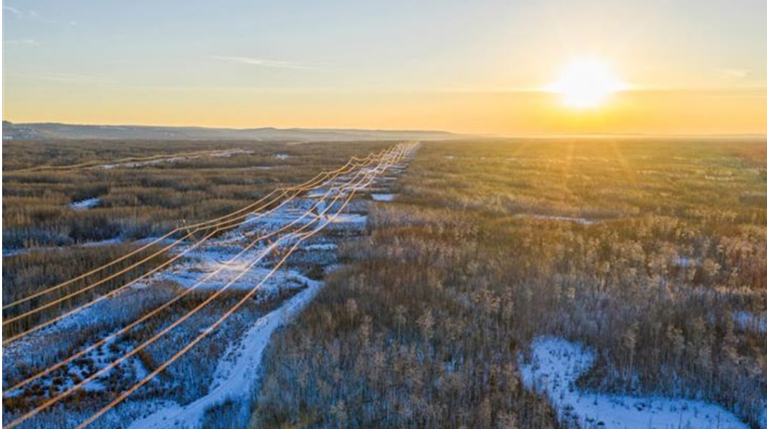
Figure A-22 The 500kV Transmission Line Right of Way Above the Site C Dam (January 2026)
