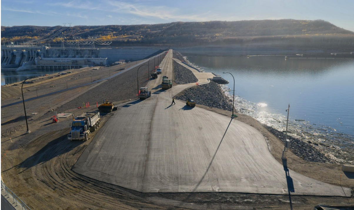
Figure A-3 Dam Crest Road Paving (October 2025)
