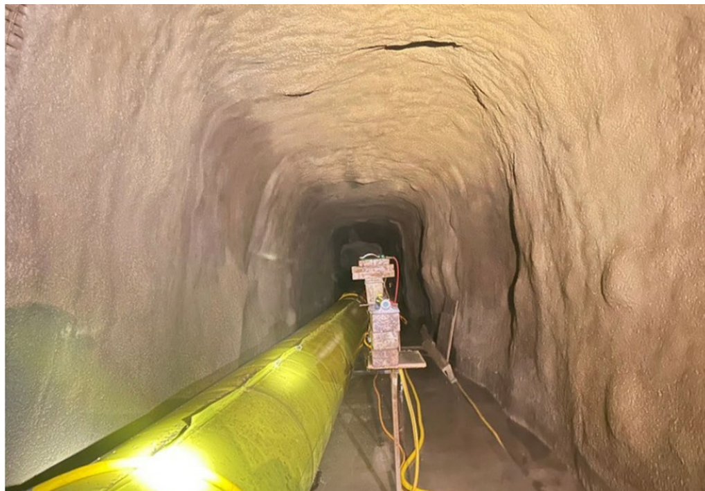
Figure A-19 Left Bank Drainage Adit: Completed Structural Enhancements (January 2026)
