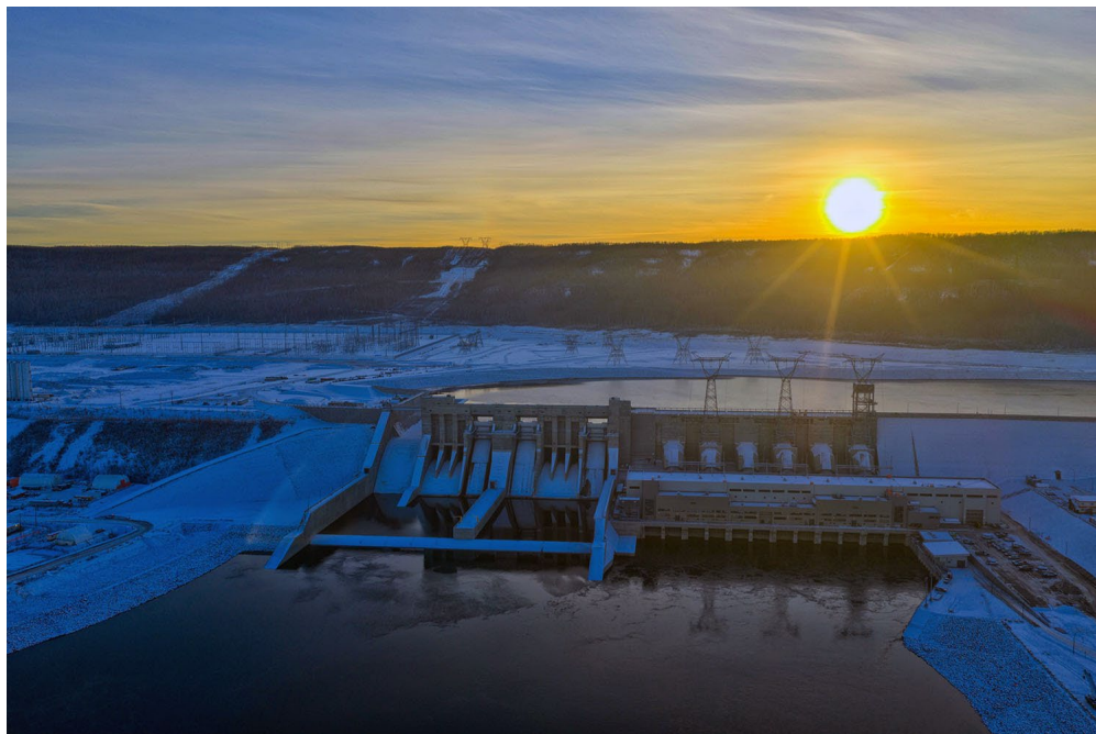
Figure A-15 Powerhouse and Generating Station (November 2025)
