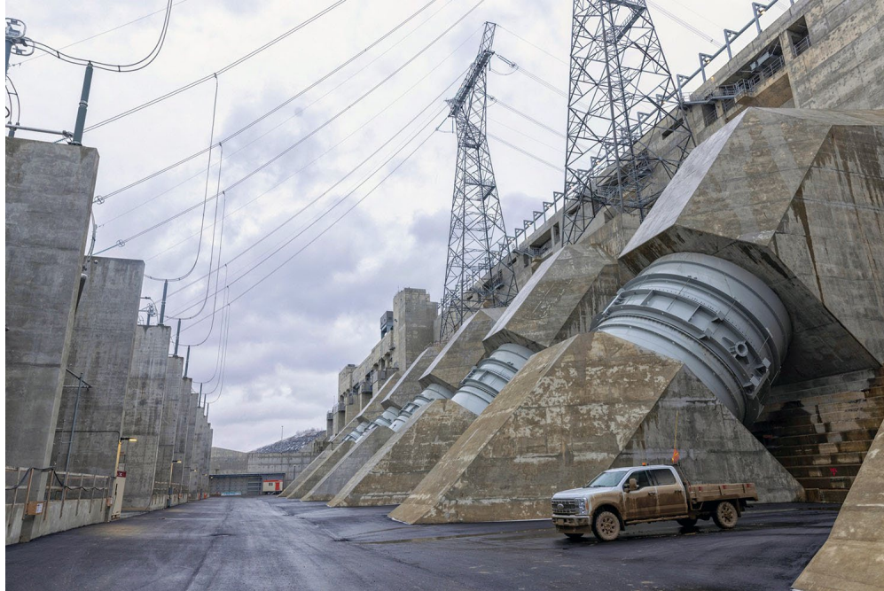
Figure A-14 Transformer Yard – Final Paving Works Complete (November 2025)
