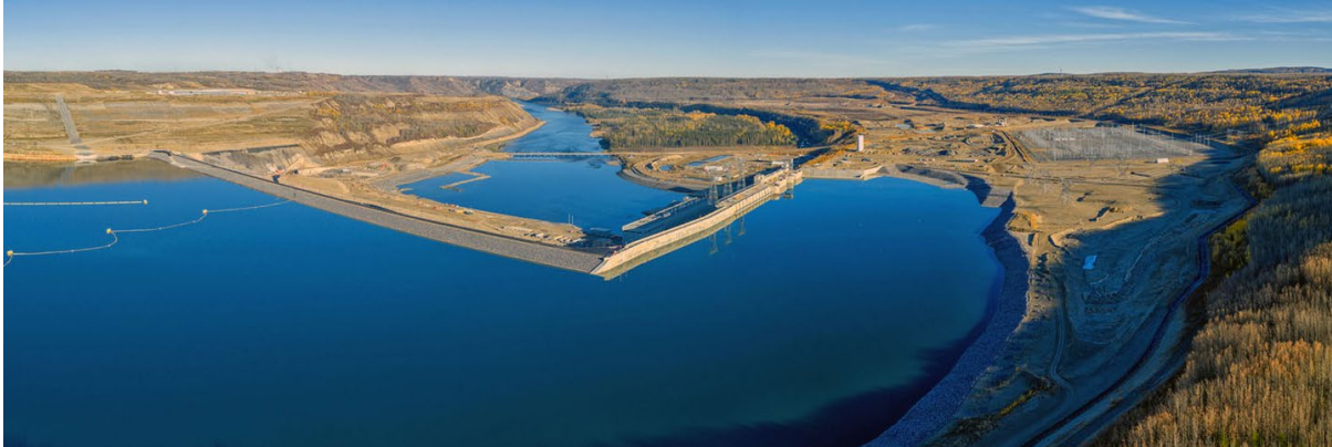
Figure A-1 Site C Dam and Generating Station (Looking Downstream) (October 2025)
