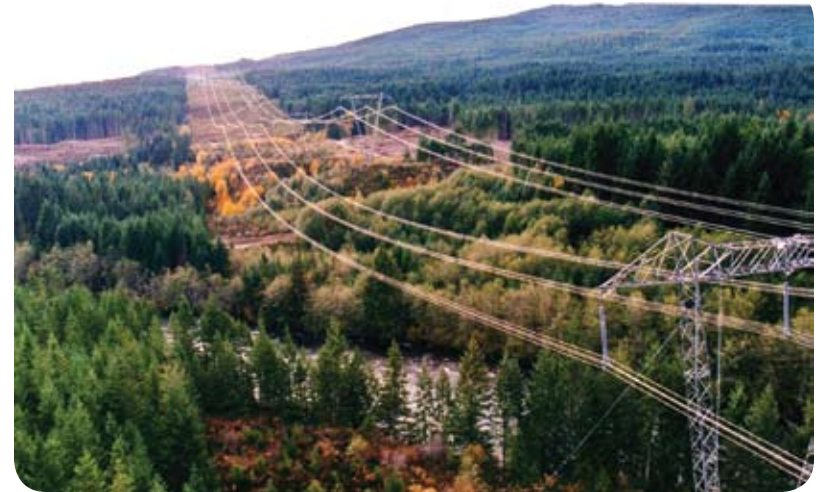
500 kv transmission lines
