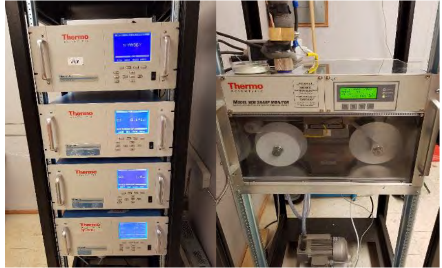
Interior: Site C North Camp
