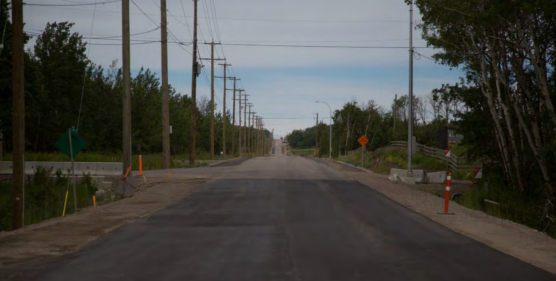
Old Fort Road Repaving and Shoulder Widening
