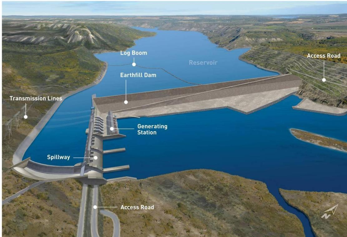
**Figure 2.1 General Arrangement of Earthfill Dam and Concrete Structures**
