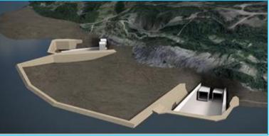
diversion tunnels, allowing a dry construction area to build the central portion of the earthfill dam. River diversion will take place in 2019, over a period of several weeks.
