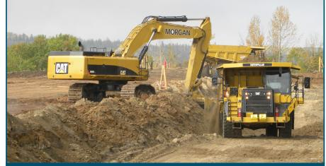
Excavation of material, part of the slope stabilization on the north bank of the Site C dam site
