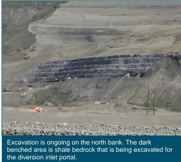
Excavation is ongoing on the north bank. The dark benched area is shale bedrock that is being excavated for the diversion inlet portal.
