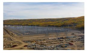
A new Site C substation has been built near the Site C dam on the south side of the Peace River. The substation connects the dam site to the new 500-kilovolt transmission lines and the supply to Fort St. John and Taylor.
