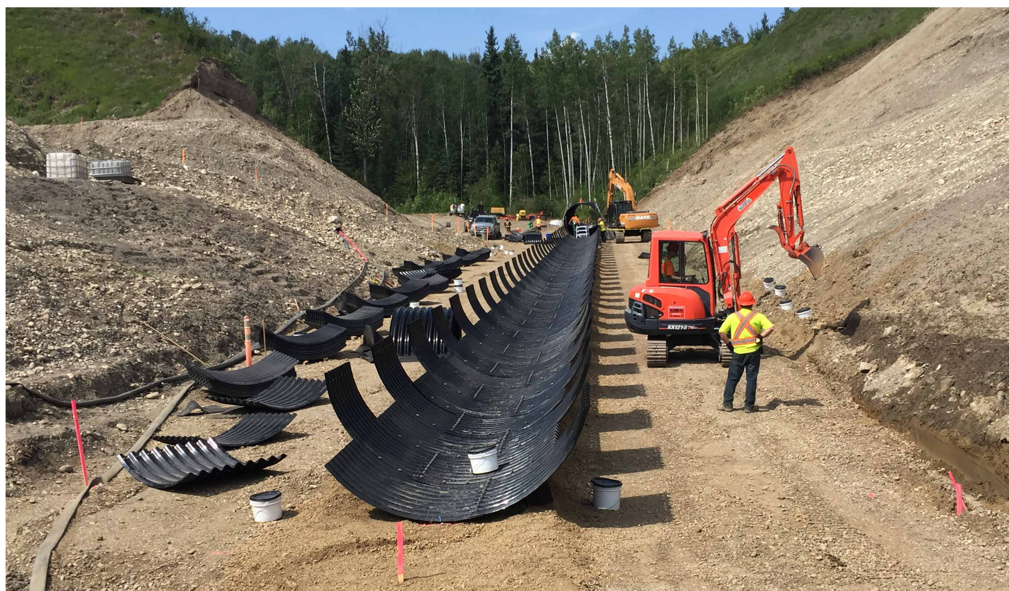
A multi-plate culvert is being installed.
