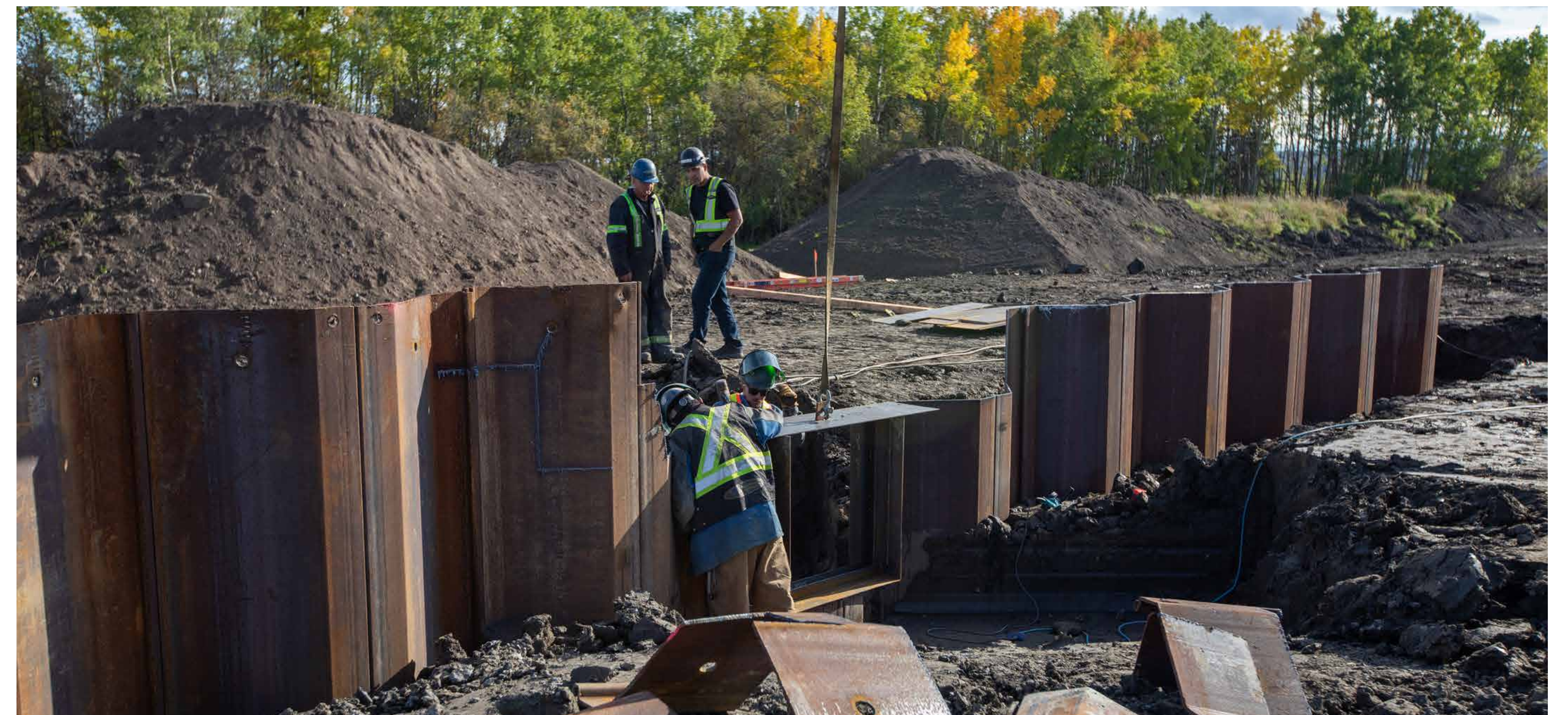
A water control structure is built.
