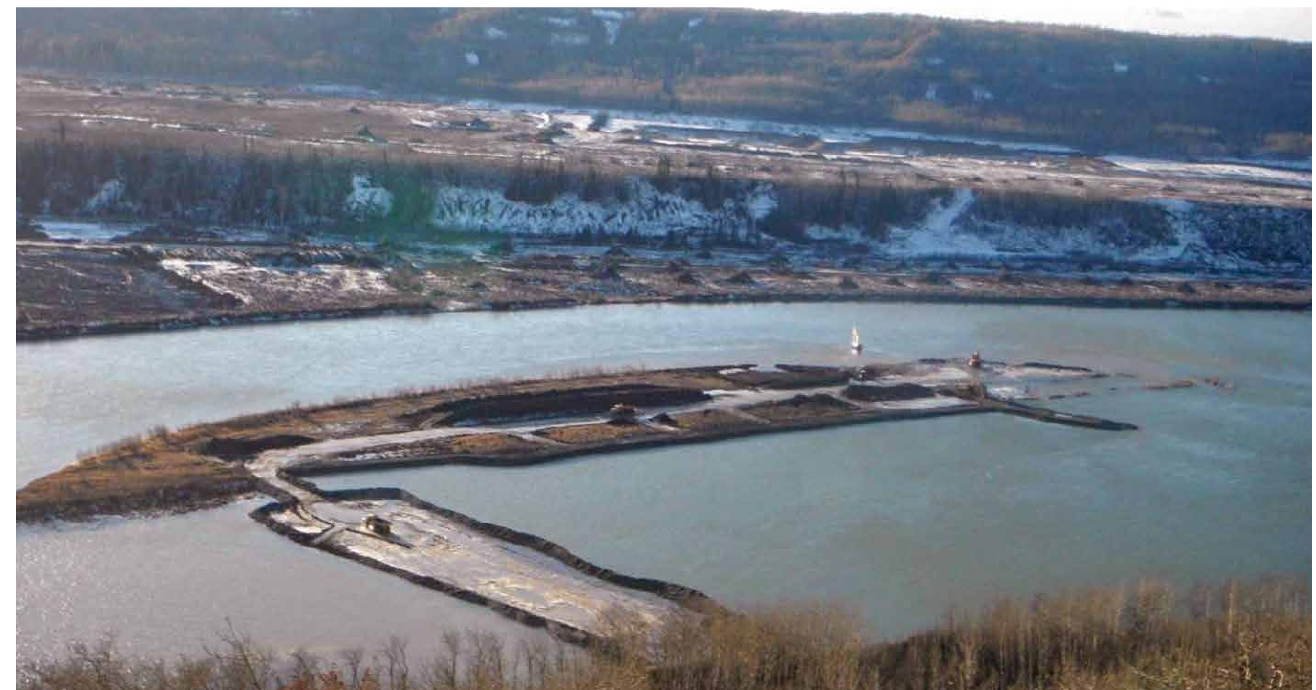
Construction of similar causeway for clearing.
