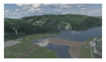
The scope of work will predominantly be constructed on a roller-compacted concrete buttress that is being constructed by Peace River Hydro Partners, as part of the main civil works contract.
