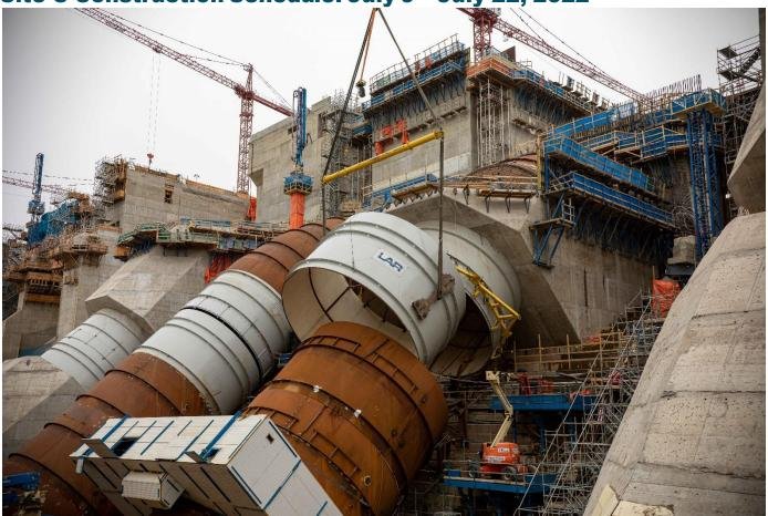
The final penstock segment is lowered into position in the powerhouse. See more photos in the <u>image</u> gallery.
