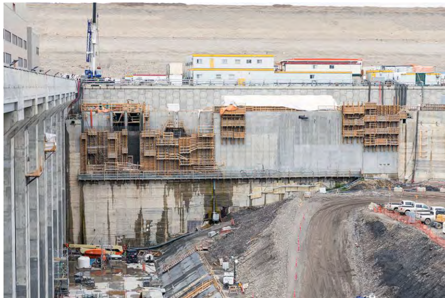
Figure A-5 Fish travelling up the Peace River will travel through the permanent upstream fish passage facility shown in this picture. Migrating fish will be sorted, tagged, and released past the dam site into the reservoir | May 2023
