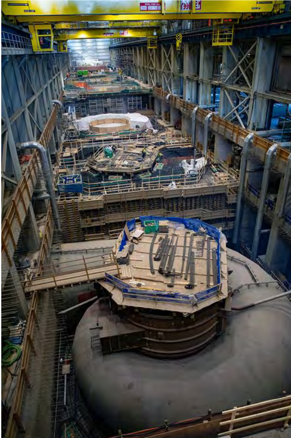
Figure A-3 Work continues in the powerhouse | April 2023
