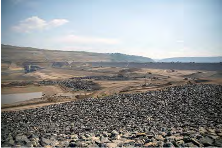
Figure A-10 Crews finish the upstream shell of the dam | June 2023
