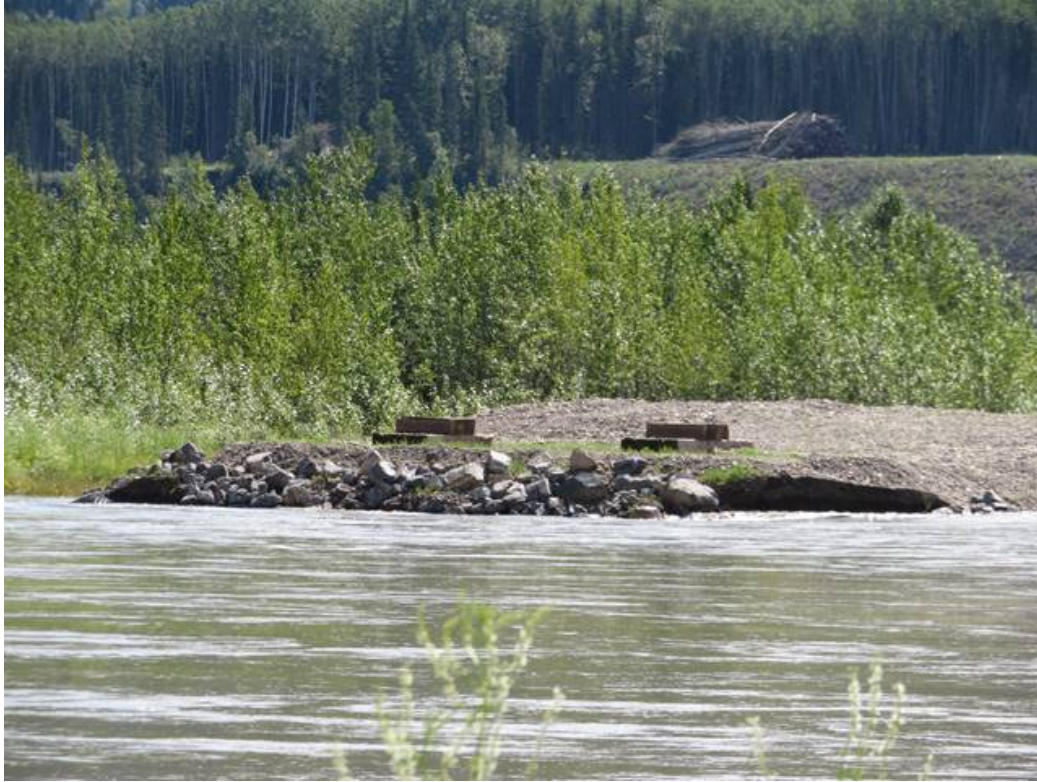
Figure 3. OLTC 16 crossing south bank abutments and causeway – to remain in place
