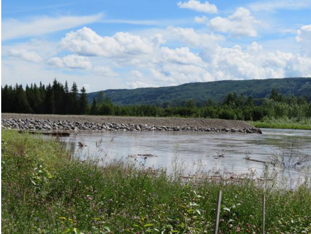
Figure 1. OLTC 16 crossing north bank causeway - to be removed
