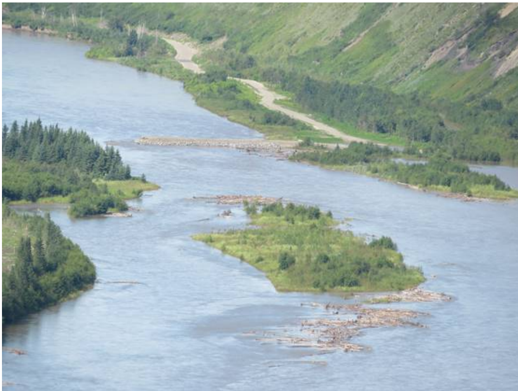
Figure 2. Aerial view of OLTC 16 crossing north bank causeway - to be removed
