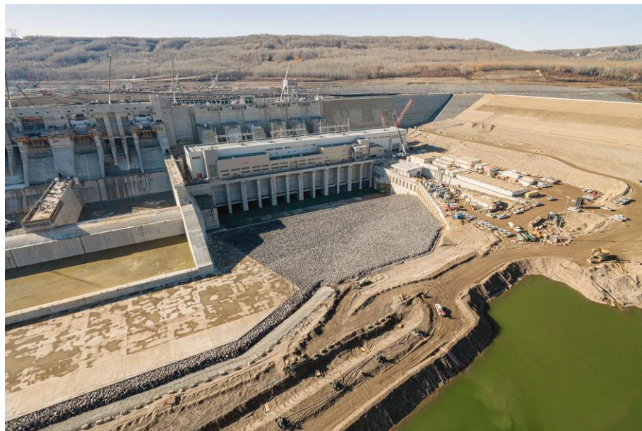
Figure A-2 Riprap placement in the tailrace area is complete | October 2023
