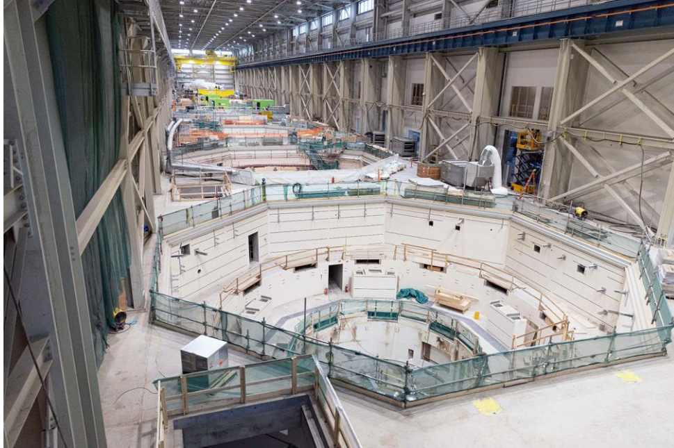
Figure A-12 The stator and rotor have been installed for the unit 3 generator | December 2023
