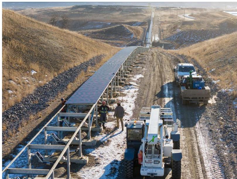
Figure A-8 Workers dismantle the five-kilometre-long till conveyor | November 2023
