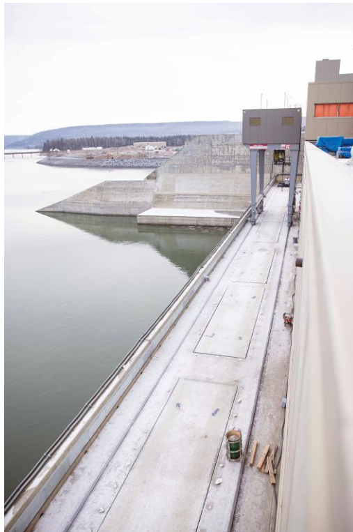
Figure A-10 The tailrace gantry crane is on rail tracks to enable it to move along the tailrace deck to access all of the draft tube maintenance gates. There are a total of 12 gates, each weighing about 40 tonnes | December 2023
