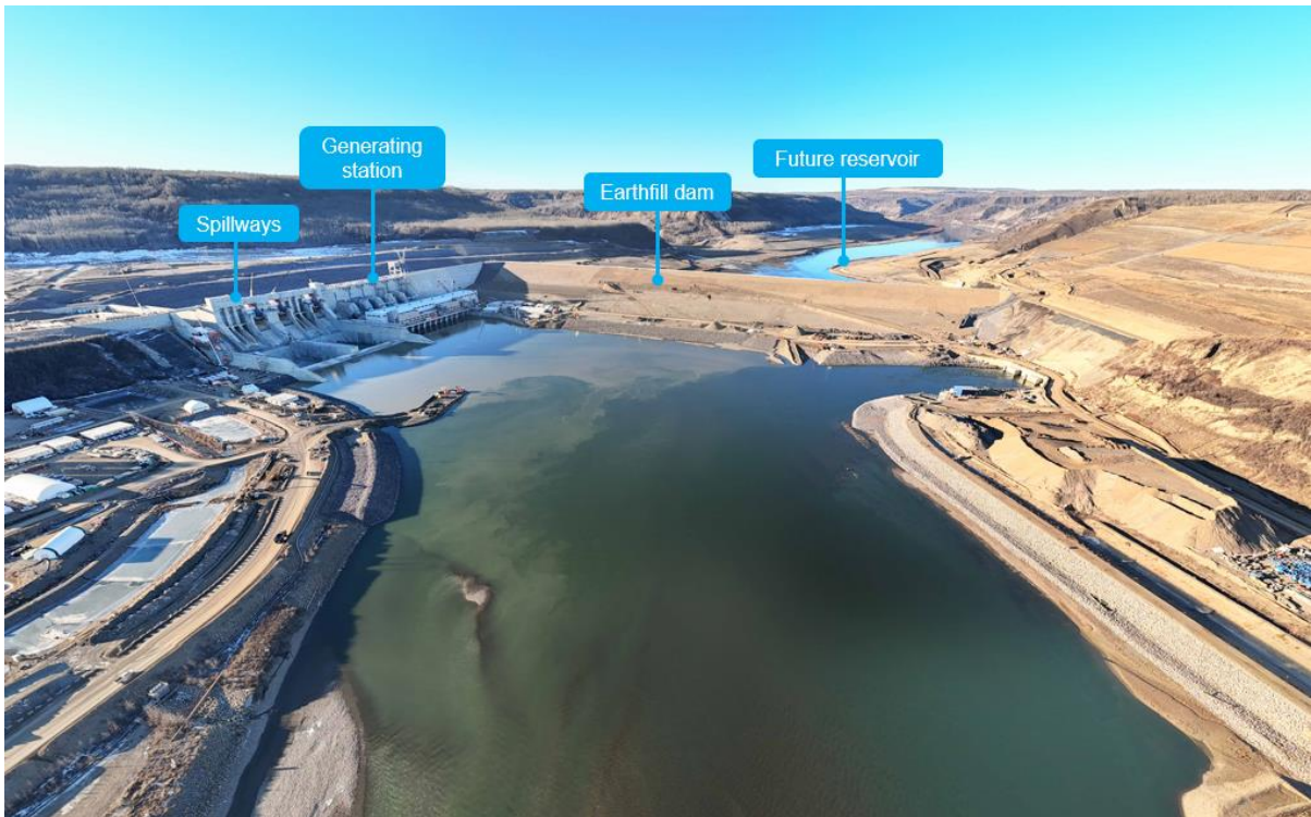
The Site C dam site (as seen in late November 2023).
