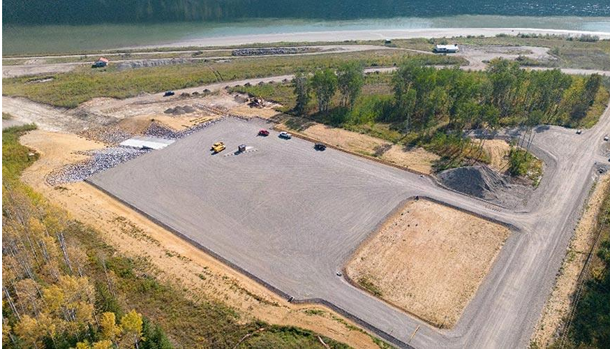
The future Lynx Creek boat launch on August 28, 2024.
