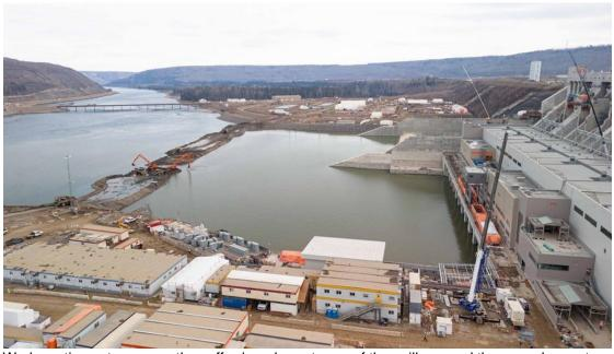
Work continues to remove the cofferdam downstream of the spillway and the powerhouse to equalize the water level on the downstream side of the dam. See more photos in our gallery.
