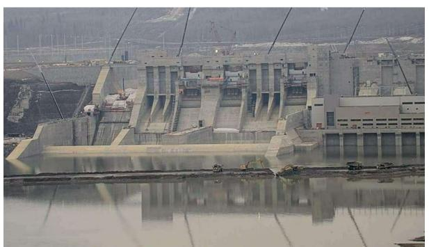
We've started to remove the cofferdam downstream of the spillway. <u>See more construction photos in</u> our gallery.
